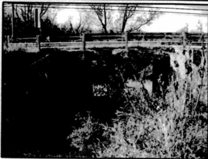
Photo 2: Culvert over Mill Creek
