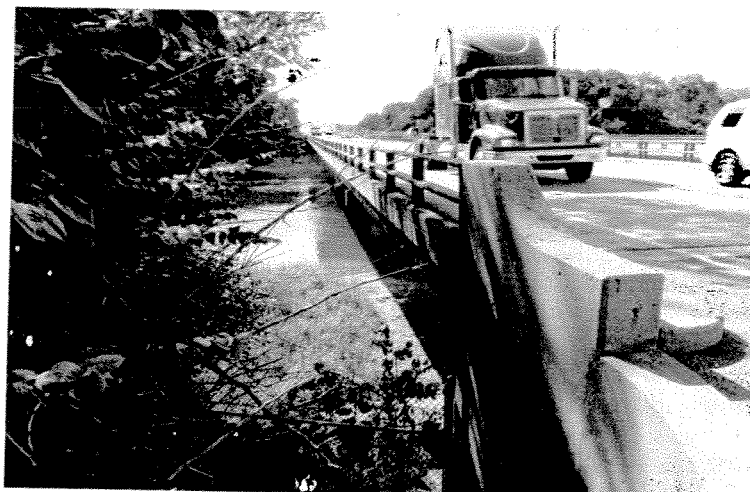
Eastbound Structure over the East Channel
