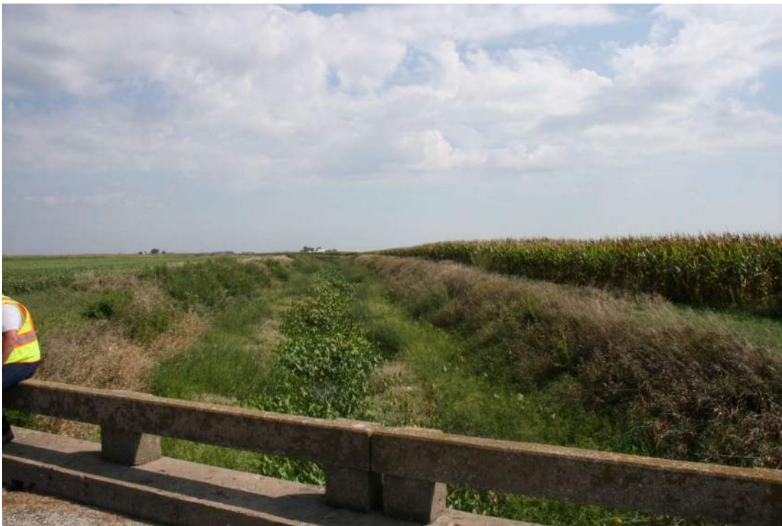
Looking East at Downstream Channel
