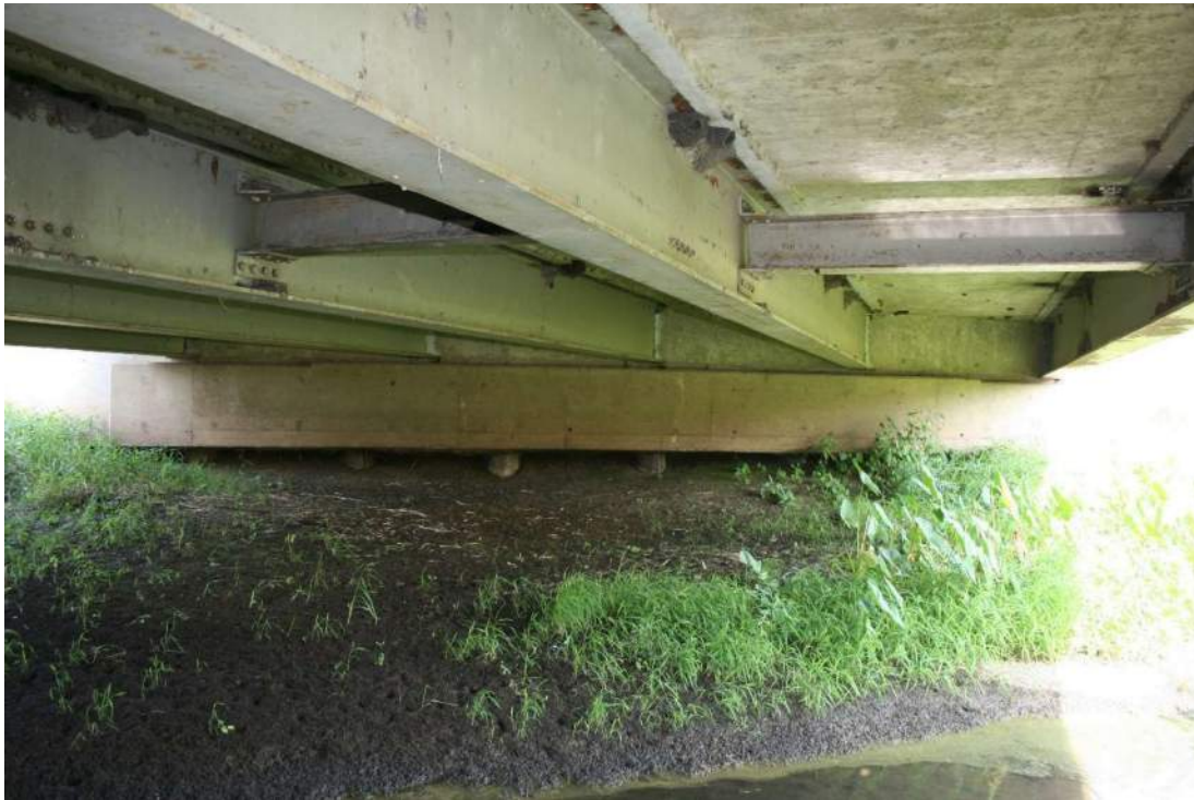
Looking North at North Abutment
