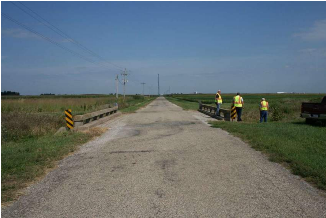
Looking North Across Existing Bridge
