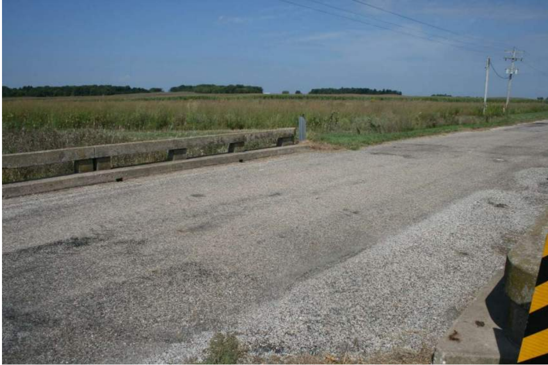
Existing Bridge Deck Surface
