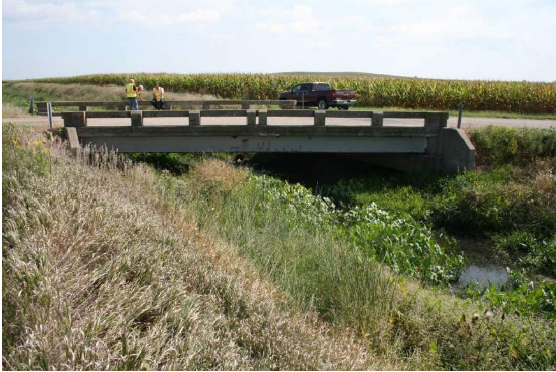
Looking East at Upstream Opening / Face of Existing Bridge
