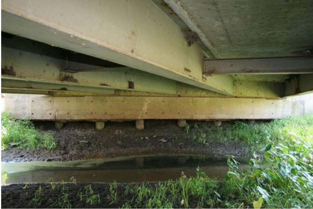
Looking South at South Abutment
