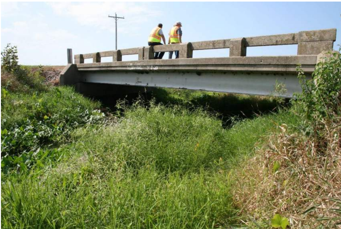
Looking Southwest at Downstream Opening / Face of Existing Bridge
