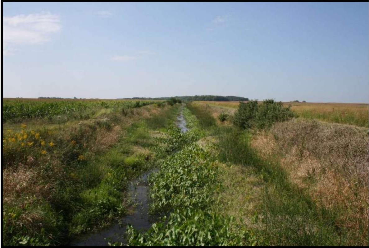
Mason County Highway 11 over Red Oak Ditch
