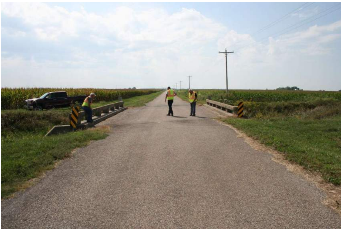
Looking South Across Existing Bridge
