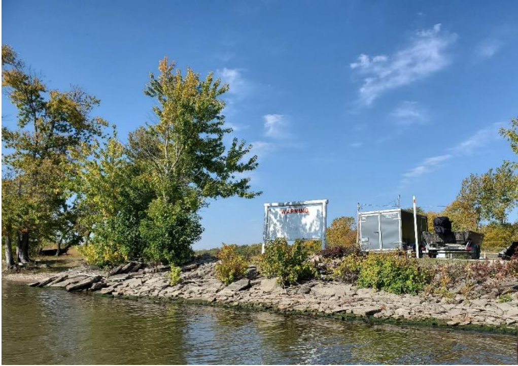
Photo 1. View of pipeline crossing looking west. Photo taken from the Mississippi River on the right descending bank.
