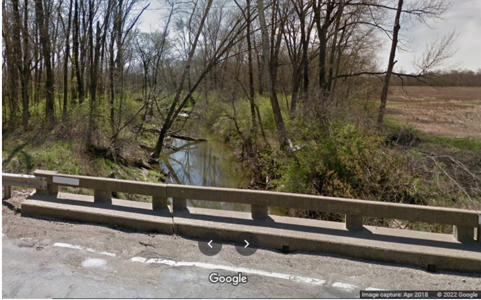
Temperature Monitoring Location at Route 1 Bridge—looking upstream
