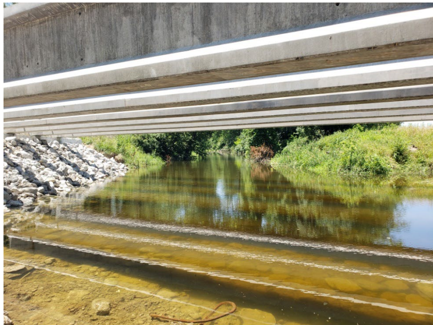
Temperature Monitoring Location at Route 1 Bridge—looking upstream
