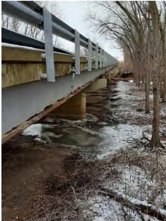
Photograph No. 14 – East Side Looking North
