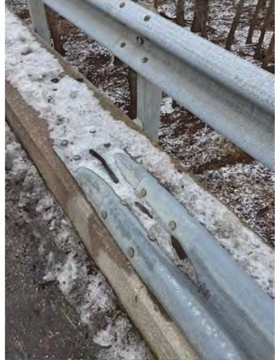
Photograph No. 11 – SE Guardrail Connection
