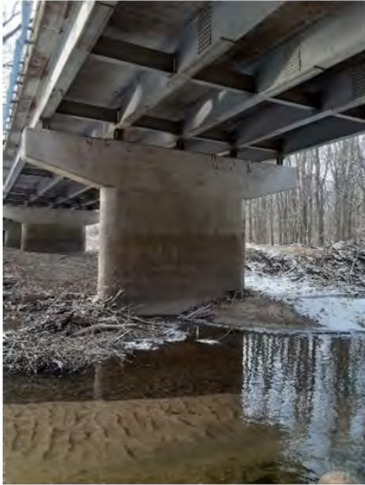
Photograph No. 9 - North Side of Pier 3
