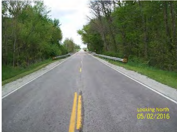
Photograph No. 1 - N 2600 East Rd (Looking North)
