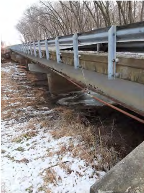
Photograph No. 10 – Bridge West Side
