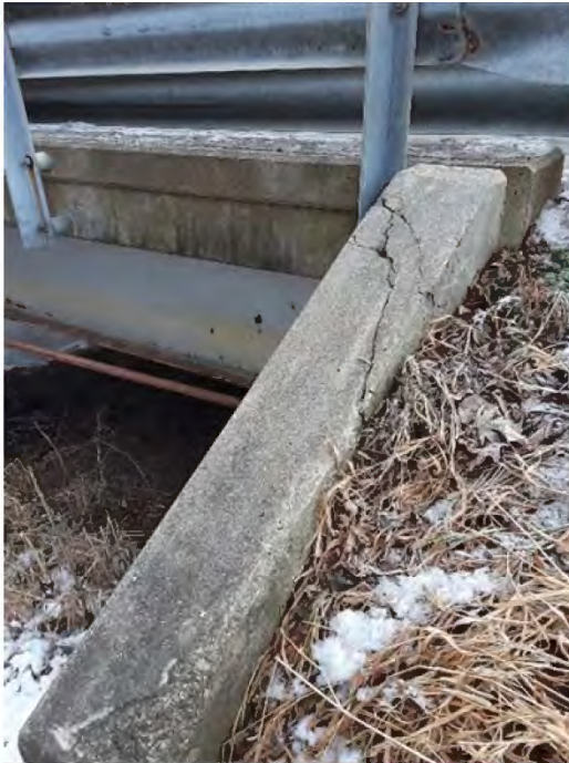
Photograph No. 6 - SW wingwall
