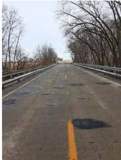
Photograph No. 3 - N 2600 East Road (Looking North)
