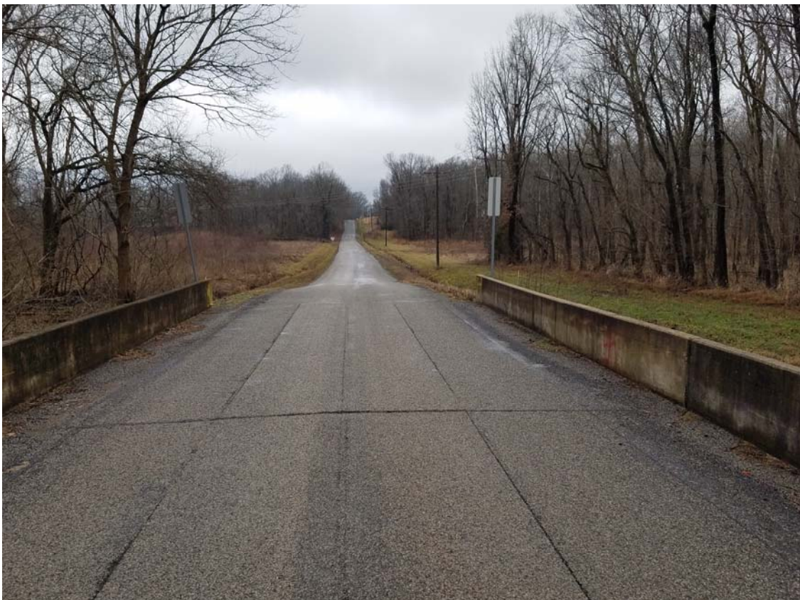
PHOTO 2 - ON BRIDGE LOOKING WEST AT WEST APPROACH
