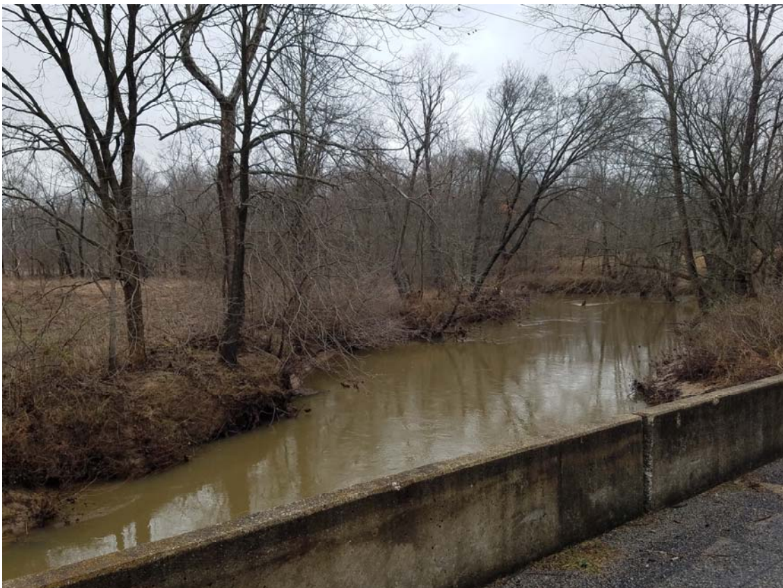
PHOTO 4 - ON BRIDGE LOOKING NORTH AT CHANNEL(DOWNSTREAM)
