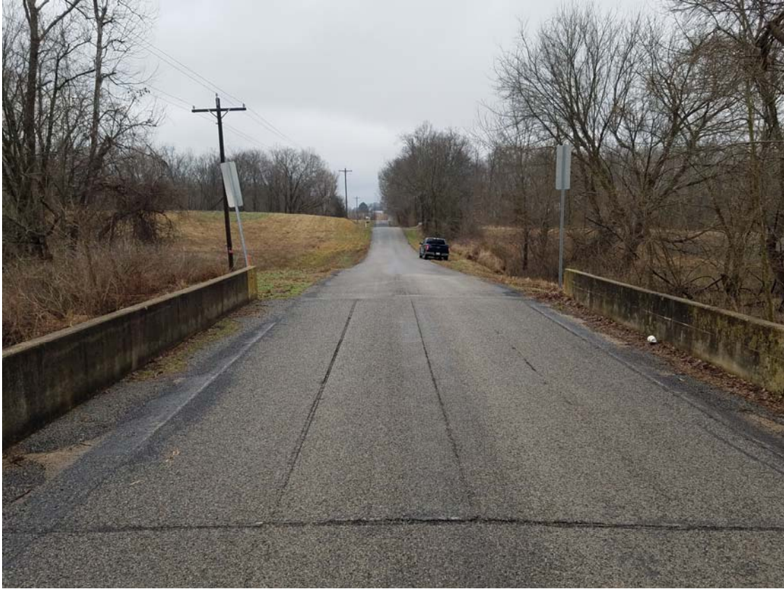
PHOTO 1 - ON BRIDGE LOOKING EAST AT EAST APPROACH
