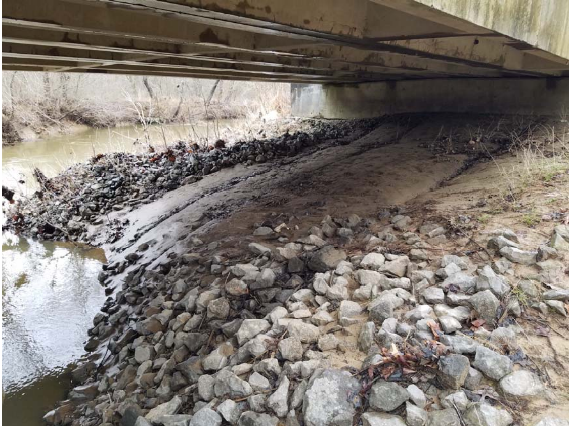
PHOTO 7 - EAST ABUTMENT AND BOTTOM OF CHANNEL BEAMS
