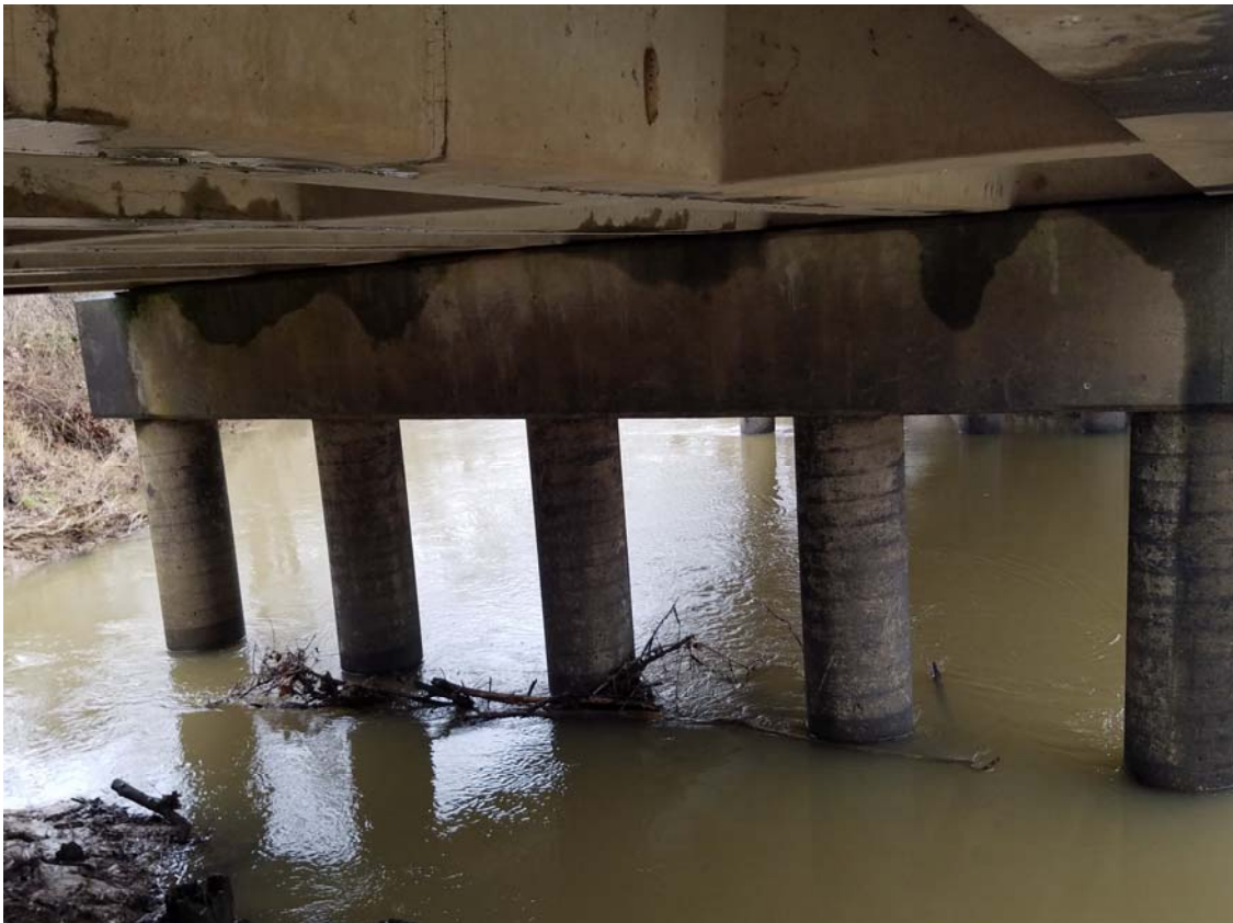
PHOTO 8 - WEST PIER AND BOTTOM OF CHANNEL BEAMS
