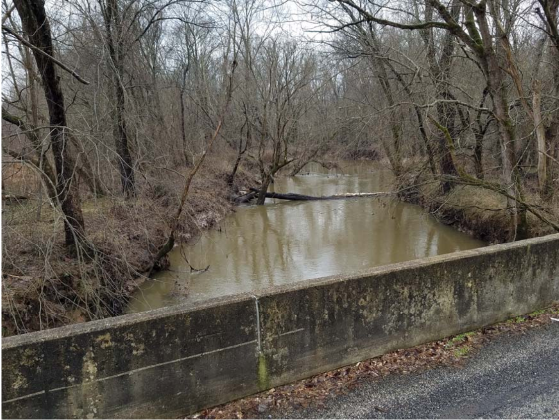
PHOTO 3 - ON BRIDGE LOOKING SOUTH AT CHANNEL(UPSTREAM)
