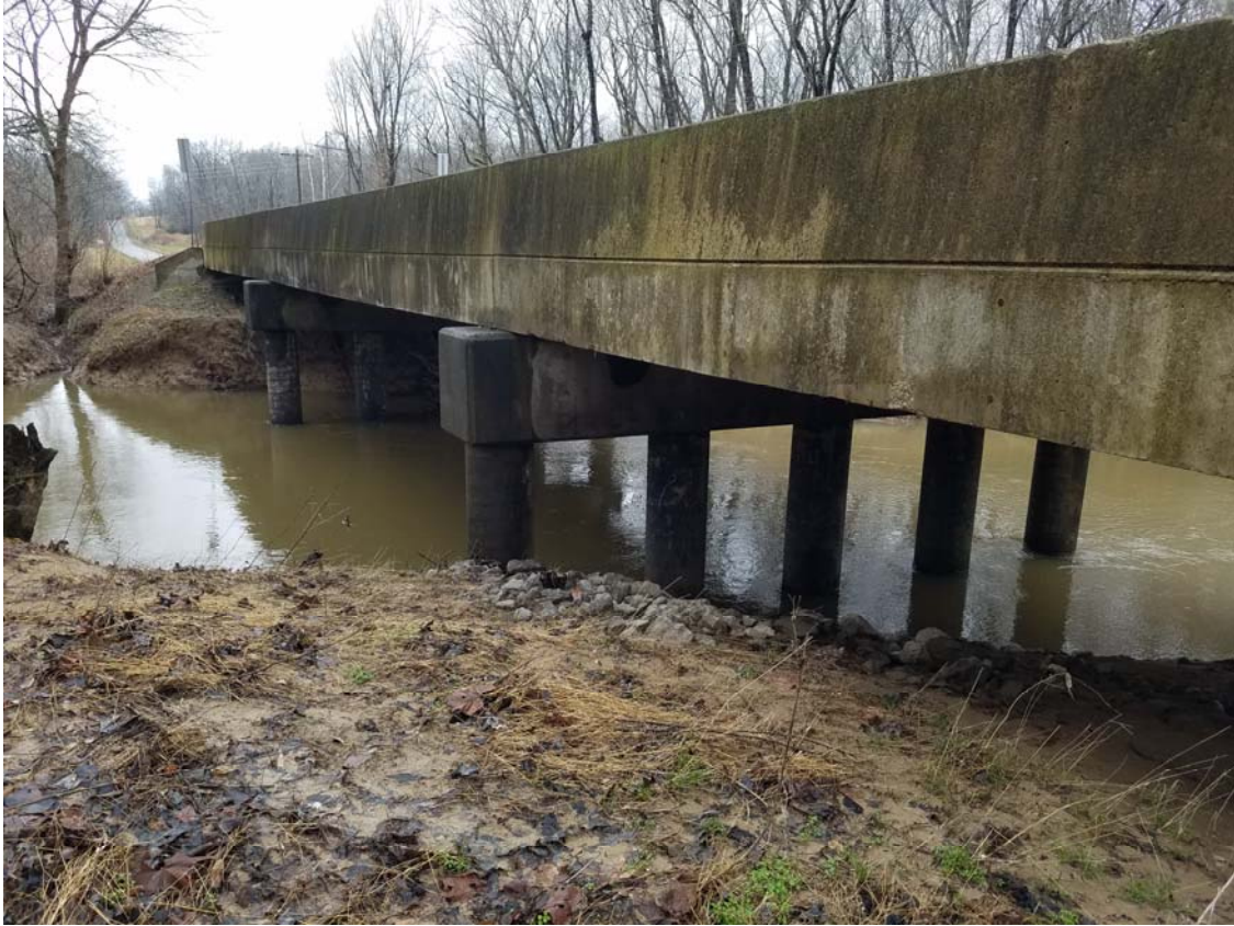
PHOTO 5 - LOOKING AT SOUTH BRIDGE FASCIA
