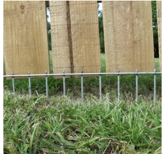
Photo 2. An example of 'No Dig' fence attachment that would be installed at the gate locations to keep turtles from entering the station under the gates.
