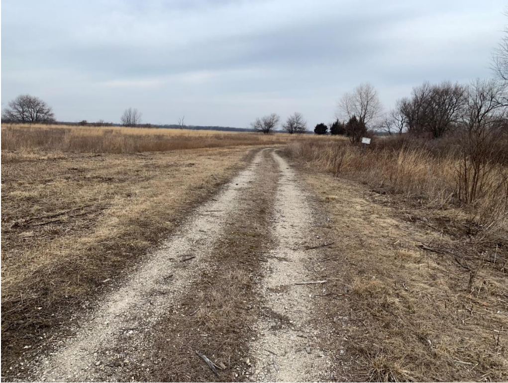
Photo 1. Entrance to the site at Heidecke Lake that will be used for access during construction. Access will be matted with timber matting. Grundy County, IL.
