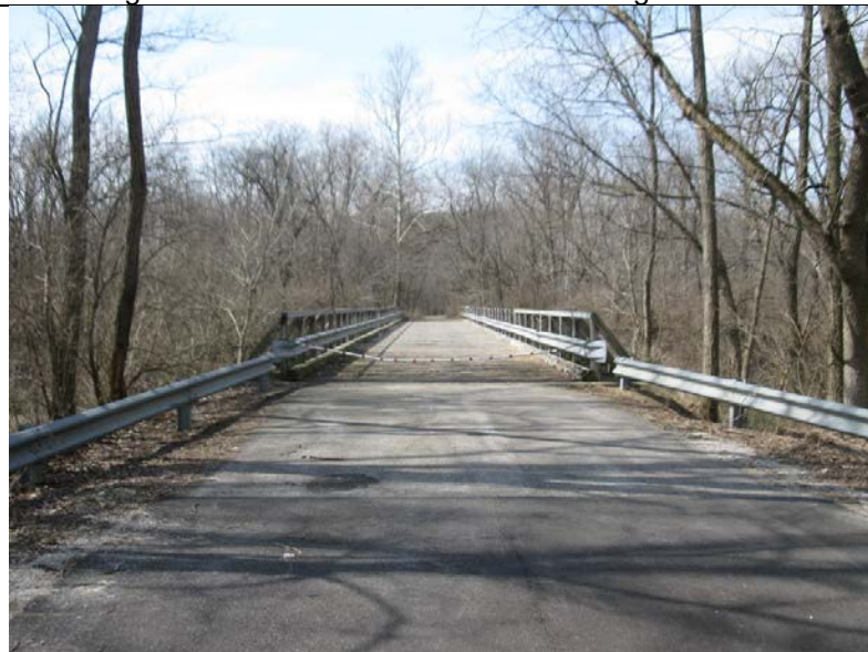
12. Looking west from east side of Pond 6 bridge.
