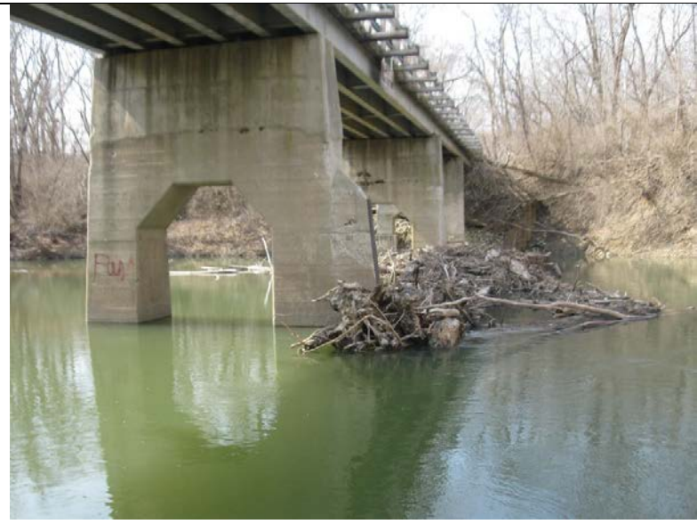
10. Facing southwest from northeast side of bridge.
