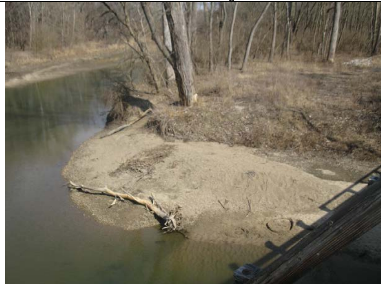
19. River bank on northeast side of bridge.
