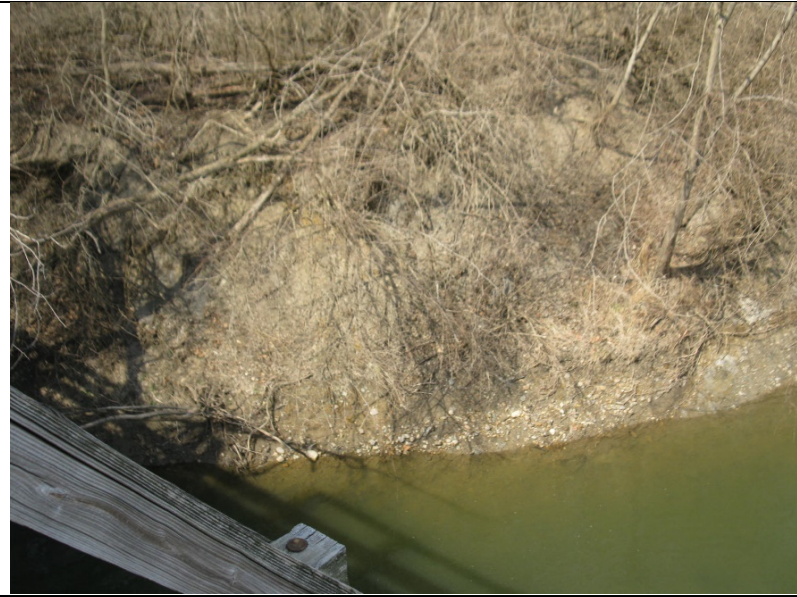
18. River bank on northwest side of bridge.
