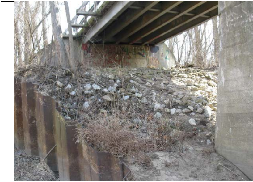
9. Facing southeast from north side of bridge.
