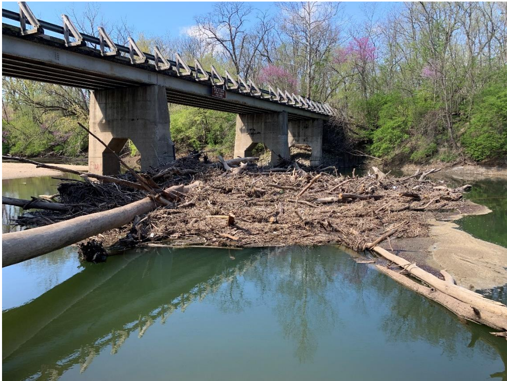
Photograph 2. Facing west towards the Pond 6 Bridge and logjam from the east bank of the Middle Fork Vermilion River.
