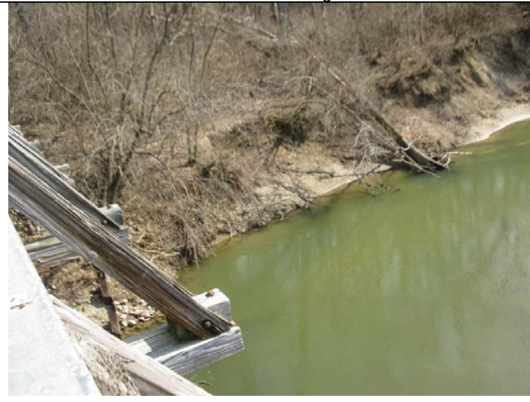
20. River bank on southeast side of bridge.
