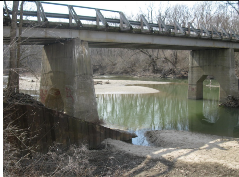
2. Looking southwest from northeast side of Pond 6 bridge.
