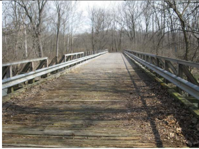
16. Facing east from top of Pond 6 bridge.
