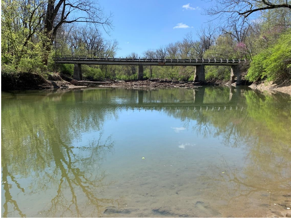
Photograph 3. Facing south towards the Pond 6 Bridge.
