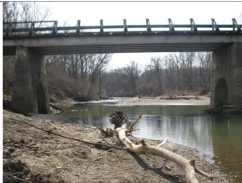
8. Facing south from northeast side of bridge.
