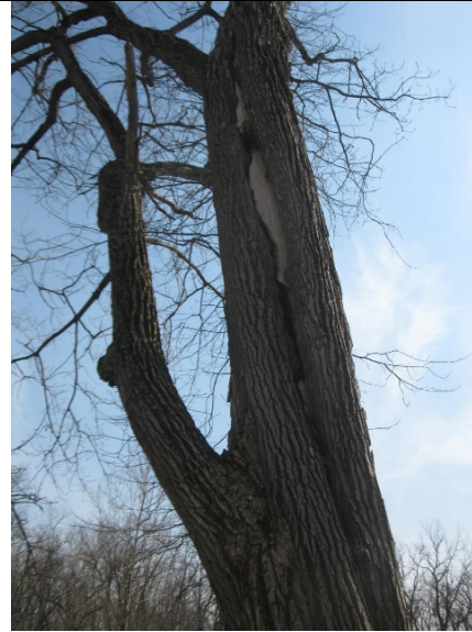
4. Tree with large crack (potential bat roosting habitat) on northeast side of bridge.
