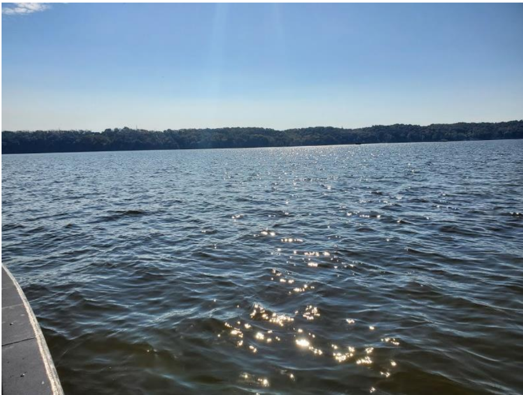
Photo 6. View facing east. Photo is looking from mid-channel towards the left descending bank over the scour area.
