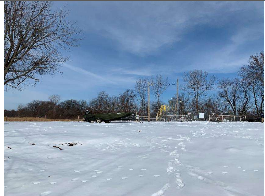
Right-of-way view from northwestern shoreline at crossing (facing northwest)
