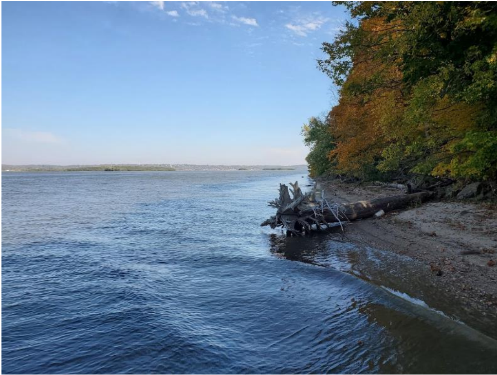
Photo 5. View facing north. Photo is of the left descending bank looking upstream of the pipeline crossing.
