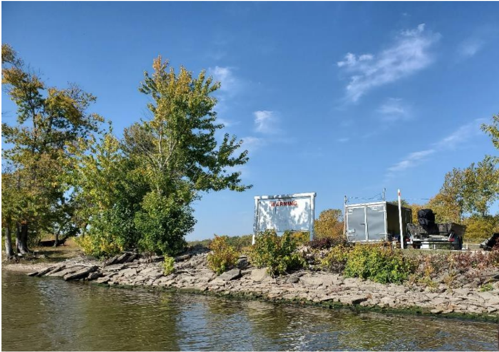
Photo 1. View of pipeline crossing looking west. Photo taken from the Mississippi River on the right descending bank.
