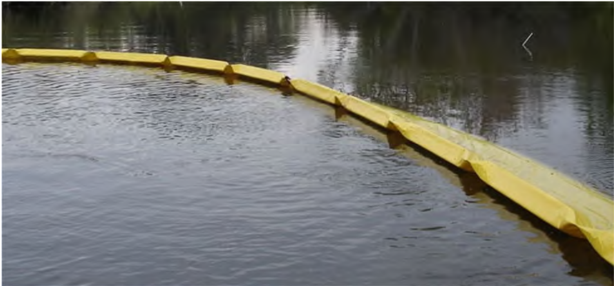
Figure 2. Example of Deployed Sediment/Turbidity Curtain in Waterway.
