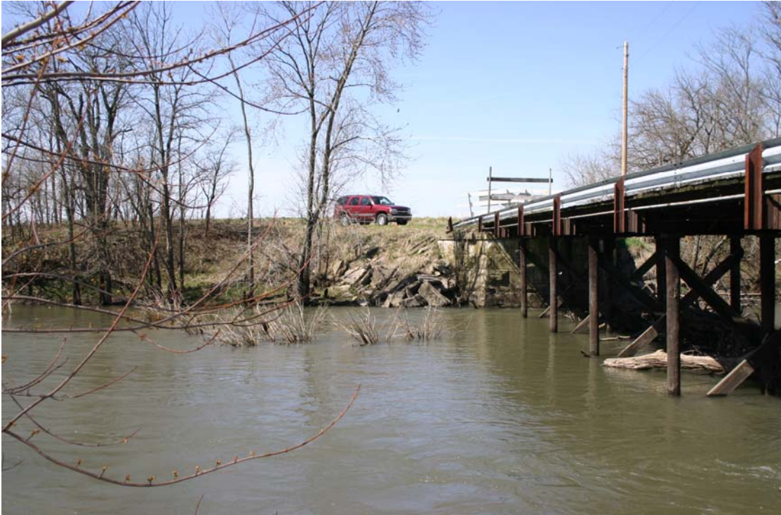
North Abutment – Looking North (Downstream side of bridge)
