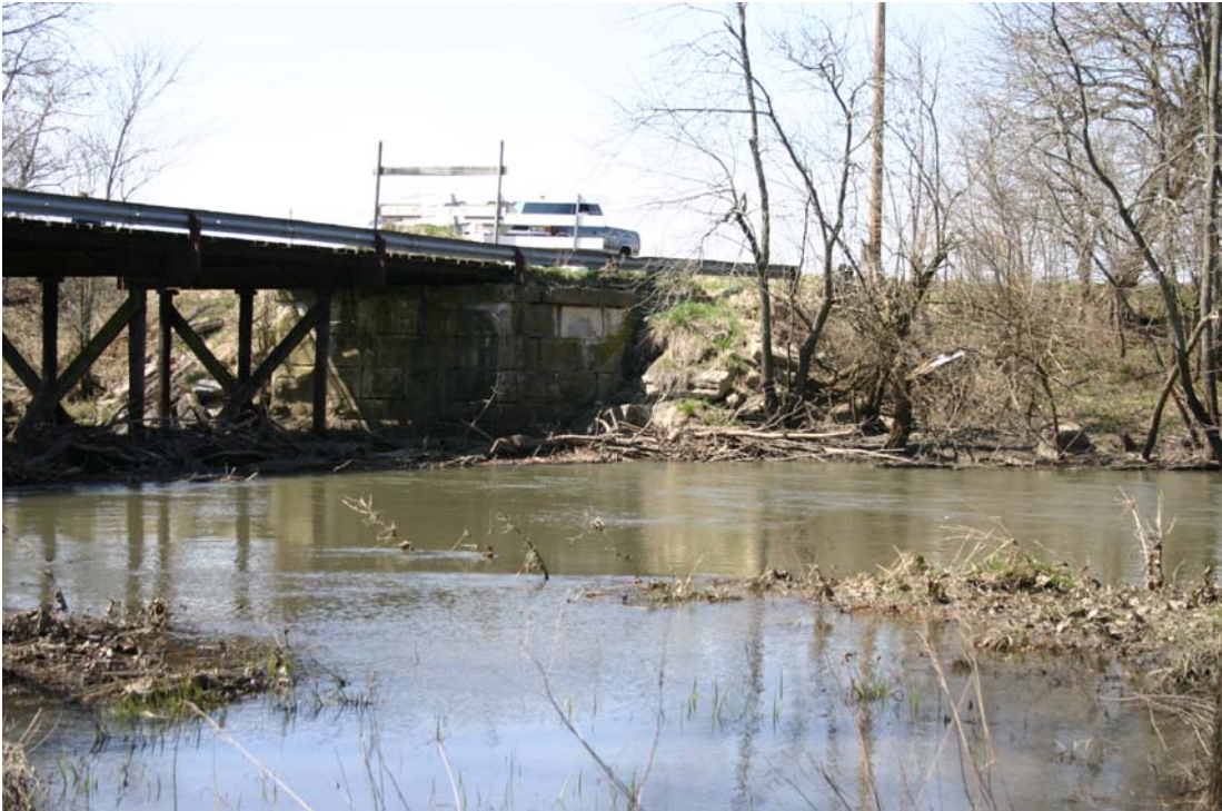
North Abutment – Looking Northwest (Upstream side of bridge)
