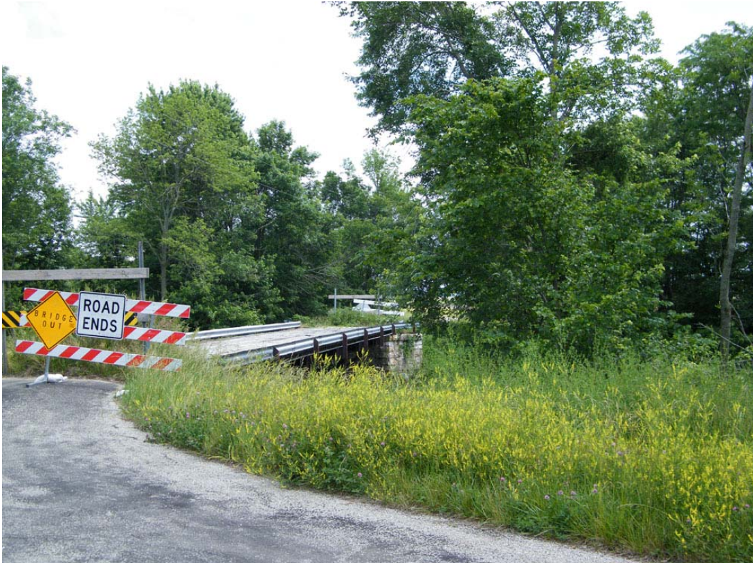
Looking southeast at north end of bridge over Brushy Fork
