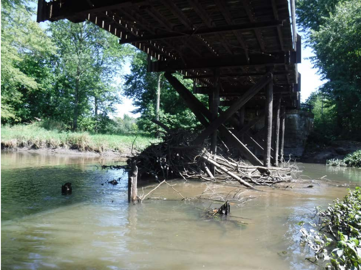
Figure 2. Woody debris accumulating along pylons of existing County Road 760N bridge (IDOT Structure No. 021-4801) over Brushy Fork in Douglas County, Illinois, on 12 August 2020. Image was taken during a survey for freshwater mussels from the north bank, facing south. Photo by A.P. Stodola, INHS.
