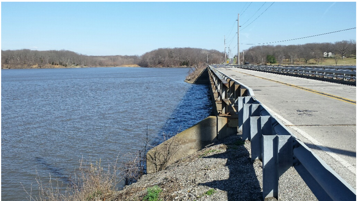
Photo 6 – Looking East Along North Side of Road from West End of West Bridge
