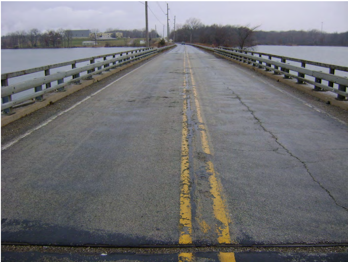
Picture 4: SN 058-3032 Top of Bridge Deck (Looking East)
