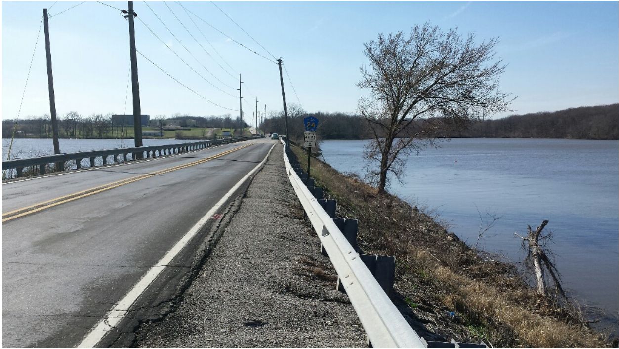
Photo 7 – Looking West Along North Side of Road from Causeway Between Bridges
