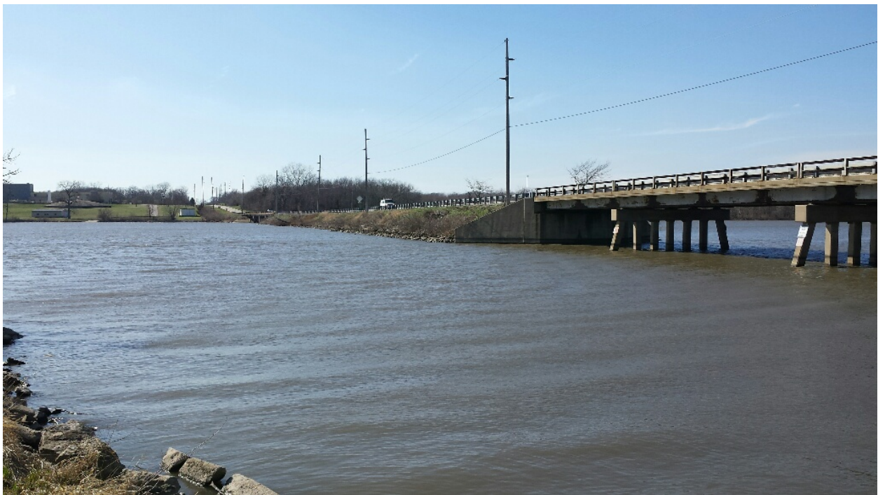
Photo 8 – Looking Northeast At Causway Between Bridges
