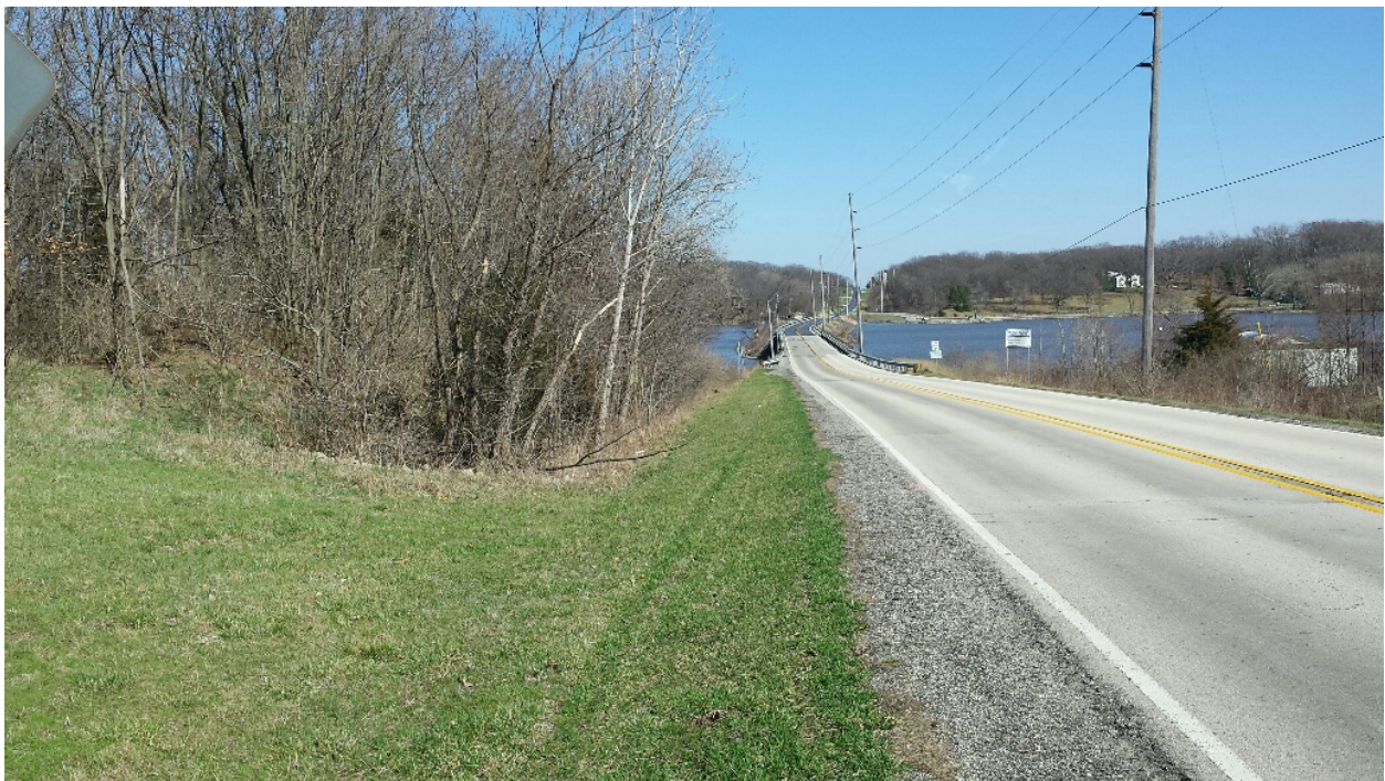
Photo 4 – Looking East Along North Side of Road West of West Bridge
