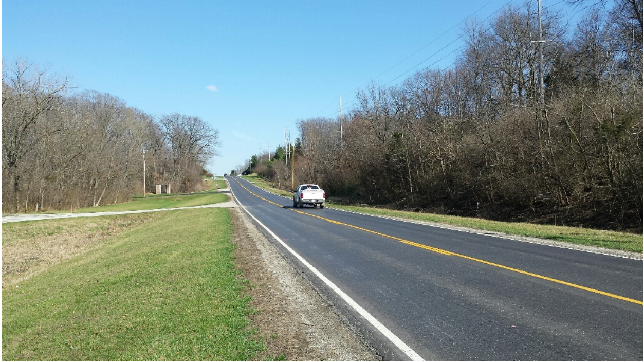
Photo 11 – Looking East Along North Side of Road at East End of Project
