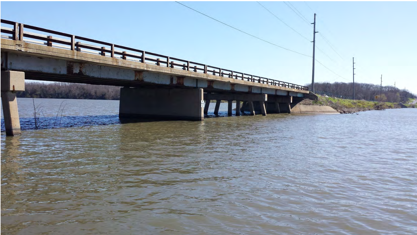
Picture 5: SN 058-3033 – Looking Northeast
