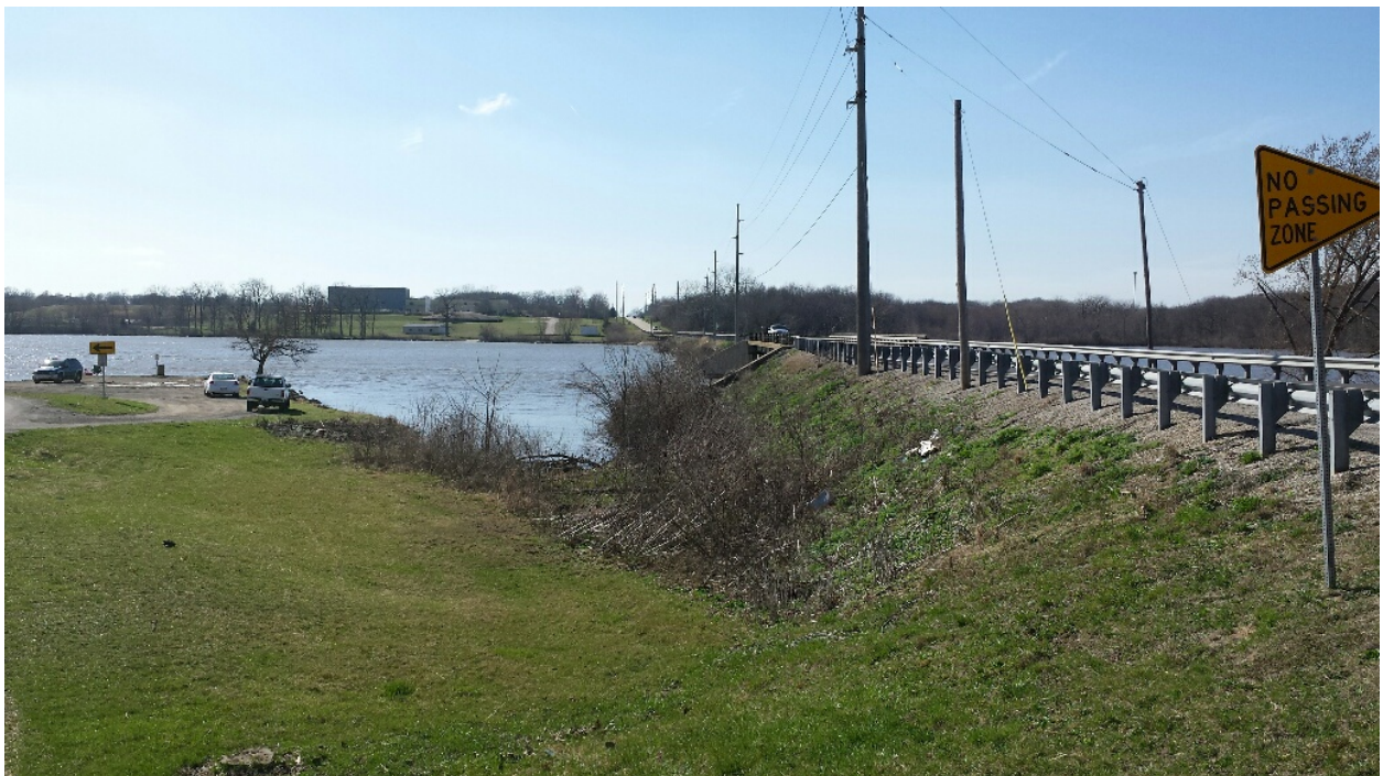
Photo 10 – Looking West Along South Side of Road from Sangamon Road
