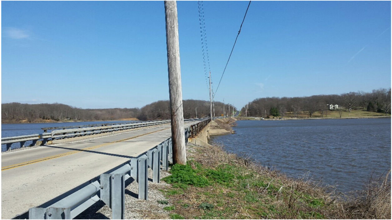
Photo 5 – Looking East Along South Side of Road from West End of West Bridge
