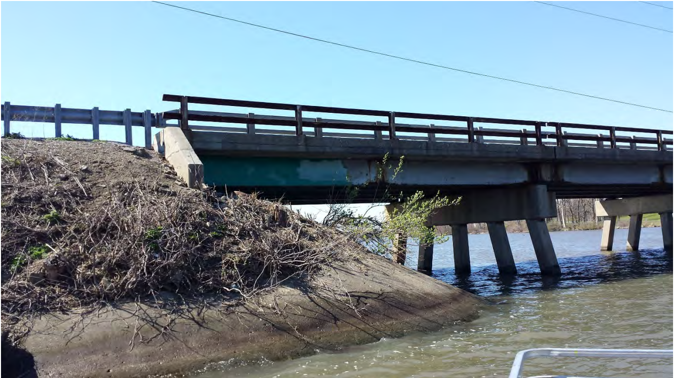
Picture 7: SN 058-3033 – East Abutment (Looking South)
