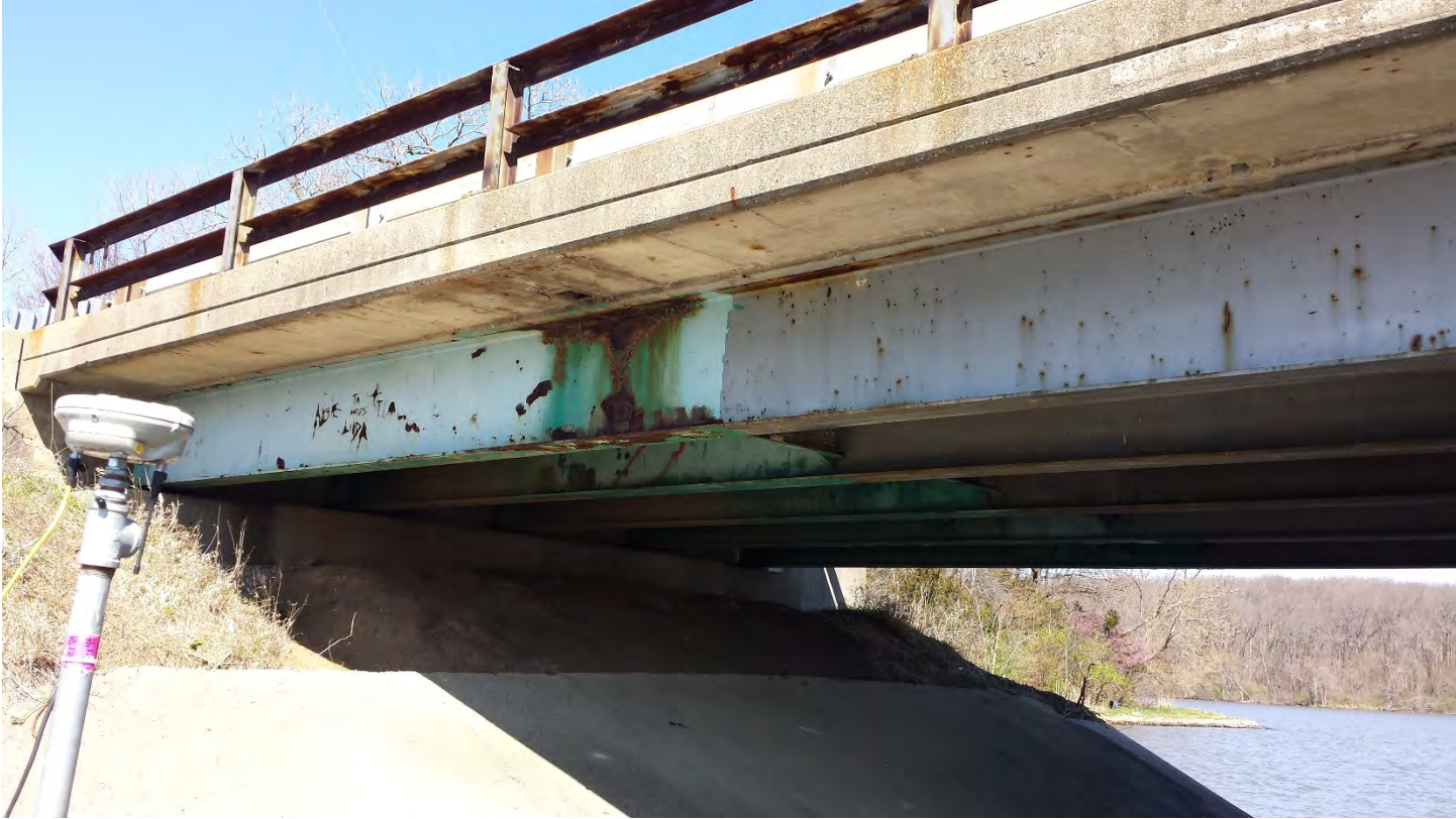
Picture 6: SN 058-3033 – West Abutment (Looking Northwest)
