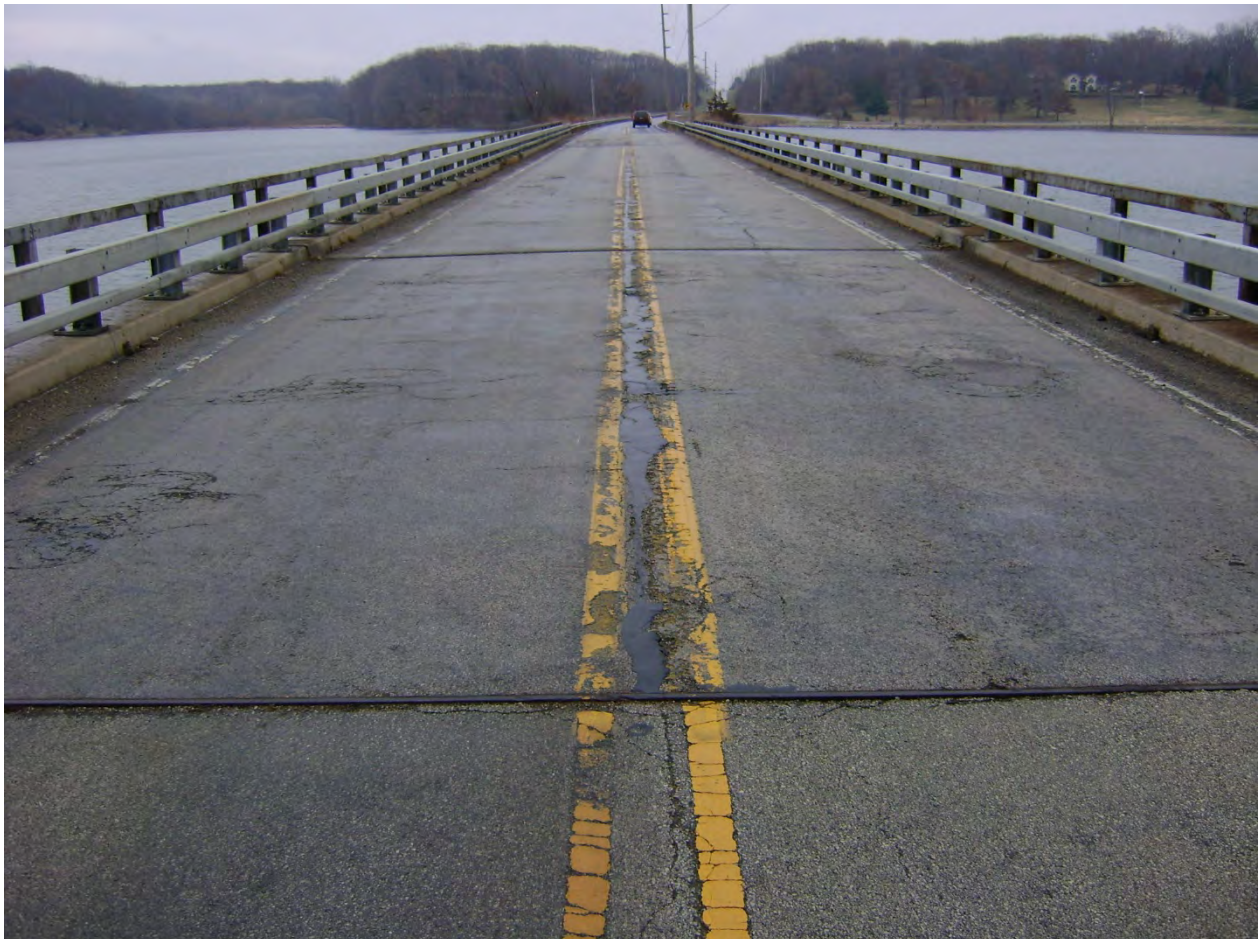
Picture 8: SN 058-3033 Top of Bridge Deck (Looking East)
