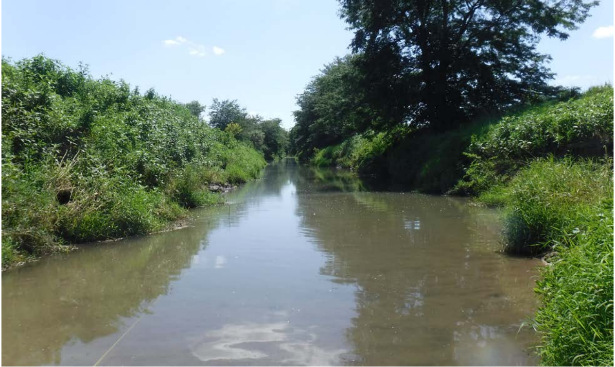
Figure 2. Middle Fork Sugar Creek from downstream of the County Highway 32/County Road 1000N (FAS 481) bridge, McLean County, Illinois, facing downstream (south) – demonstrating channelized nature of the stream – where a recipient area was established by INHS personnel on 6 August 2020. Photo by A.P. Stodola, INHS.
