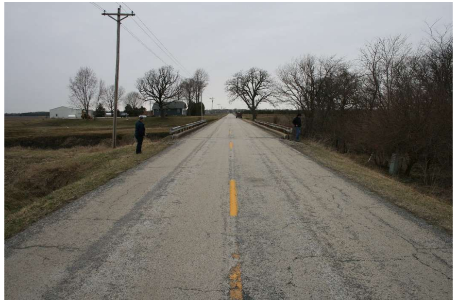
LOOKING WEST THROUGH PROJECT AREA
