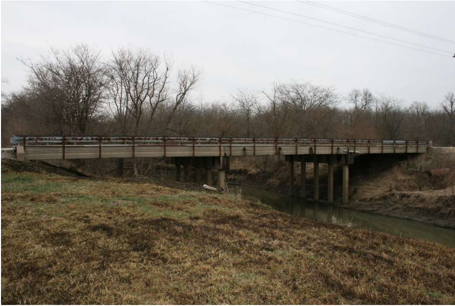
UPSTREAM OPENING – LOOKING NORTHEAST
