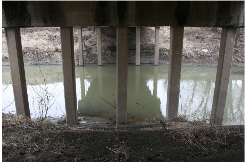
VIEW BETWEEN PIERS – LOOKING WEST
