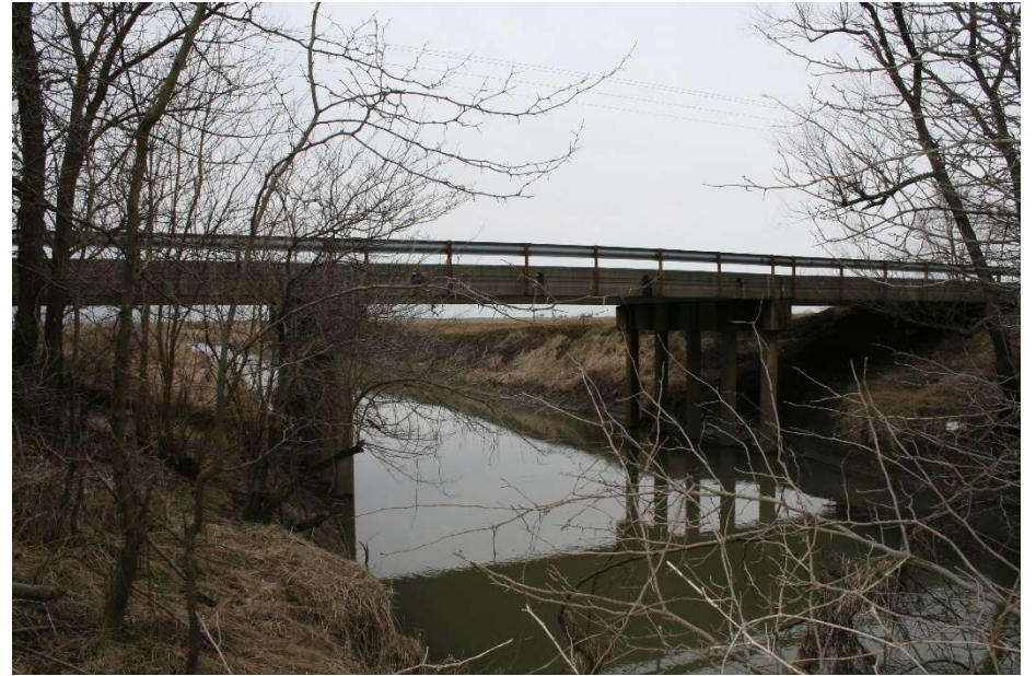
DOWNSTREAM OPENING – LOOKING SOUTHWEST
