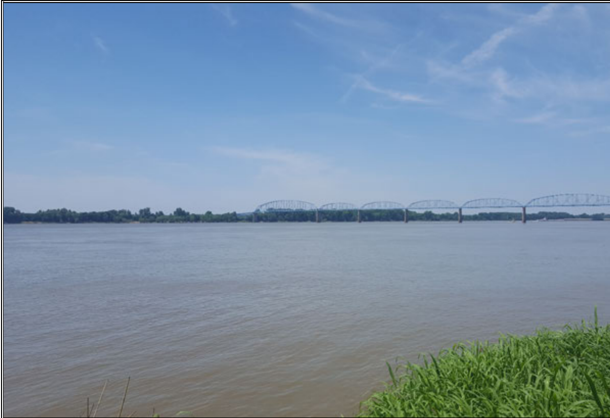
Photograph 3: View of the downstream portion of the project area, facing west from the right descending bank of the Ohio River. May 23, 2018.
