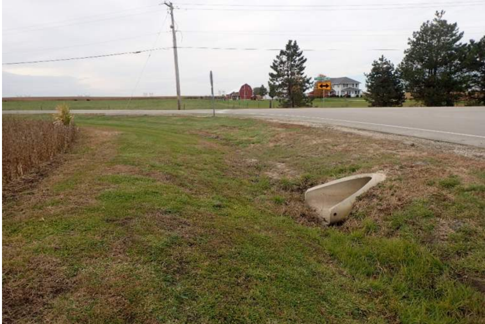
Intersection of Highpoint Road and Fox Road
