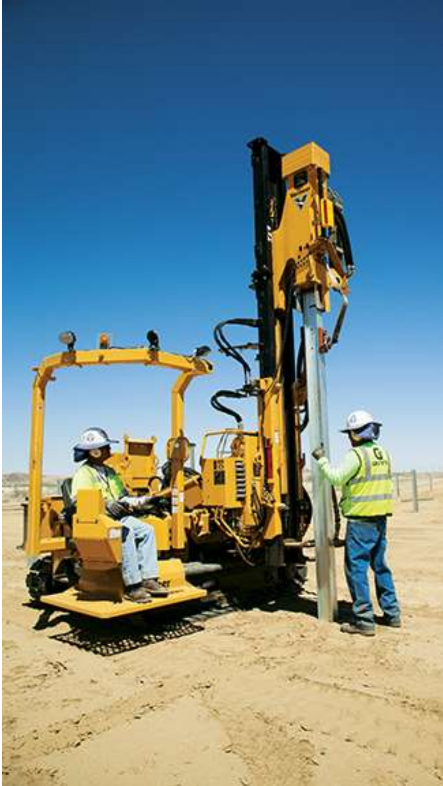
Example foundation pile driving equipment.
