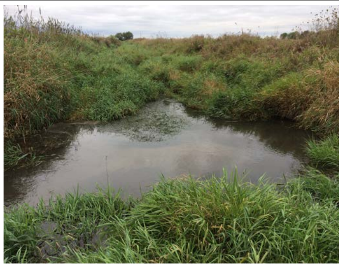
Photo 4: View from the culvert looking west downstream.
