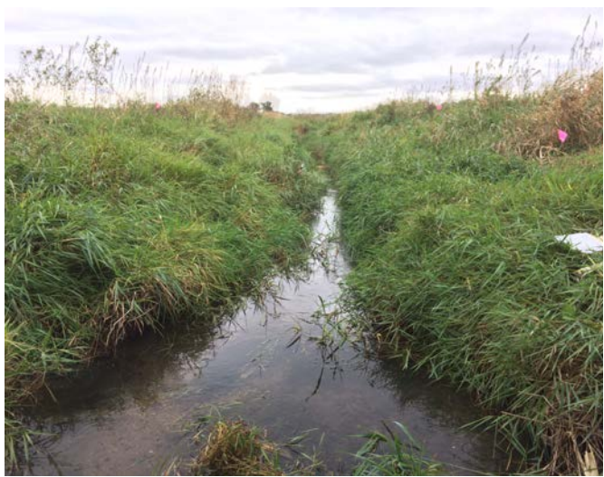
Photo 3: View from the culvert looking east upstream.
