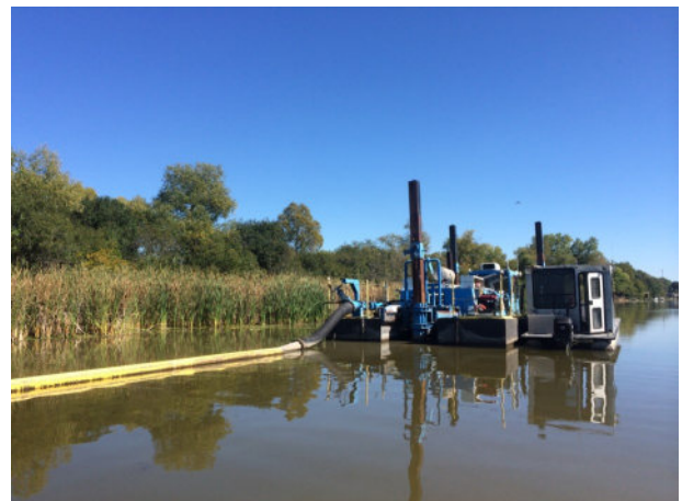
Figure 8. Fox Waterway Agency dredging a channel in Lake Marie, 2014.
