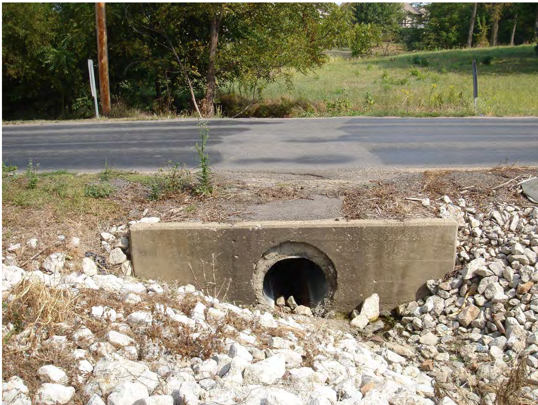
Existing culvert crossing Archer Elevator Road south of Greenbriar, looking west.
