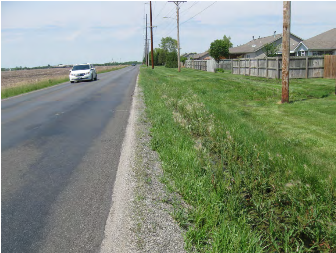
Archer Elevator road south of Hedley Road, looking north.
