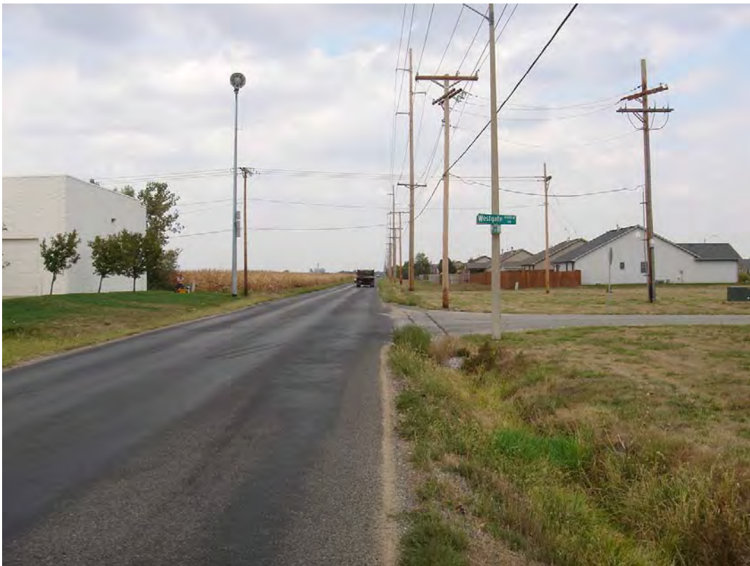
Archer Elevator Road, looking north towards Westgate Dr.
