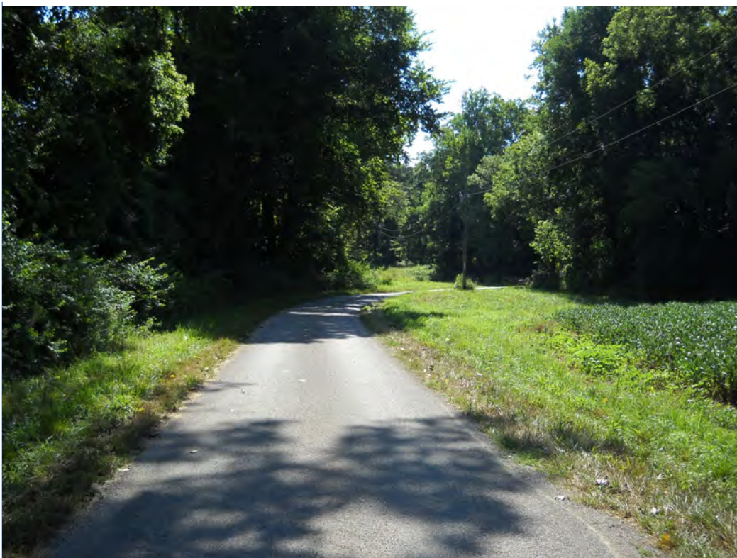
Looking easterly along Staley Road towards curves
