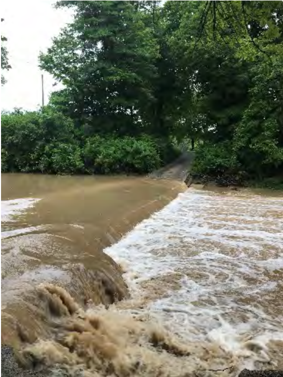
Facing northeast; downstream face of existing low water crossing (overflow culvert).
