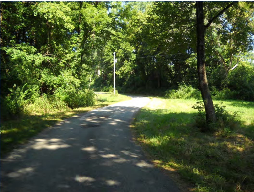
Looking westerly along Staley Road from curves east of low-water crossing
