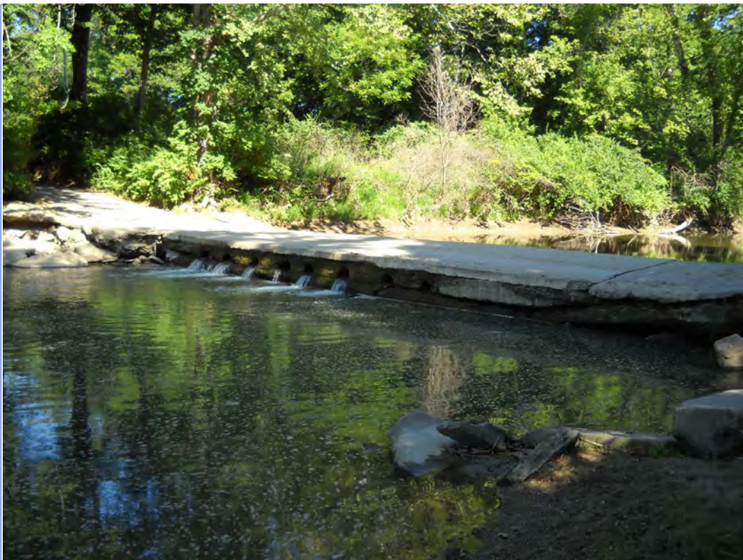
Sideview of downstream side of low-water crossing
