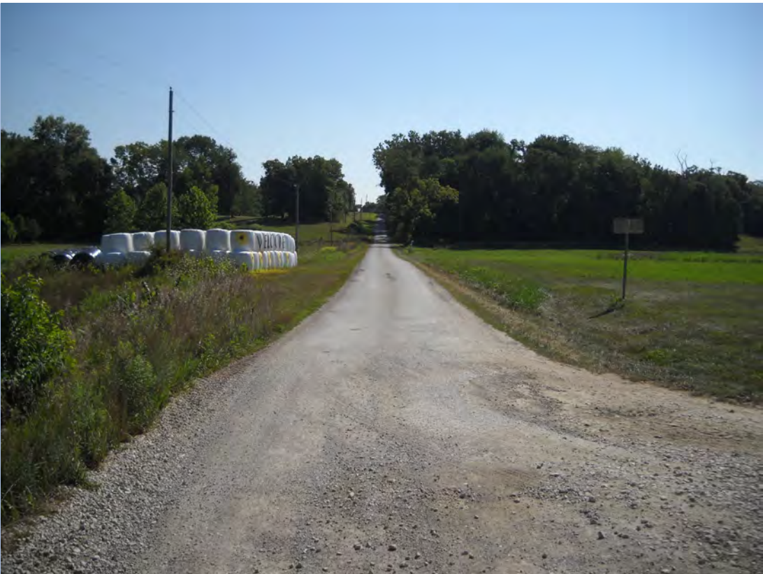
Near east end of project looking east along Staley Road
