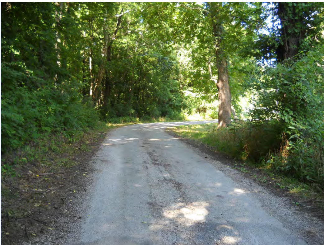
Staley Road east of low-water crossing looking west
