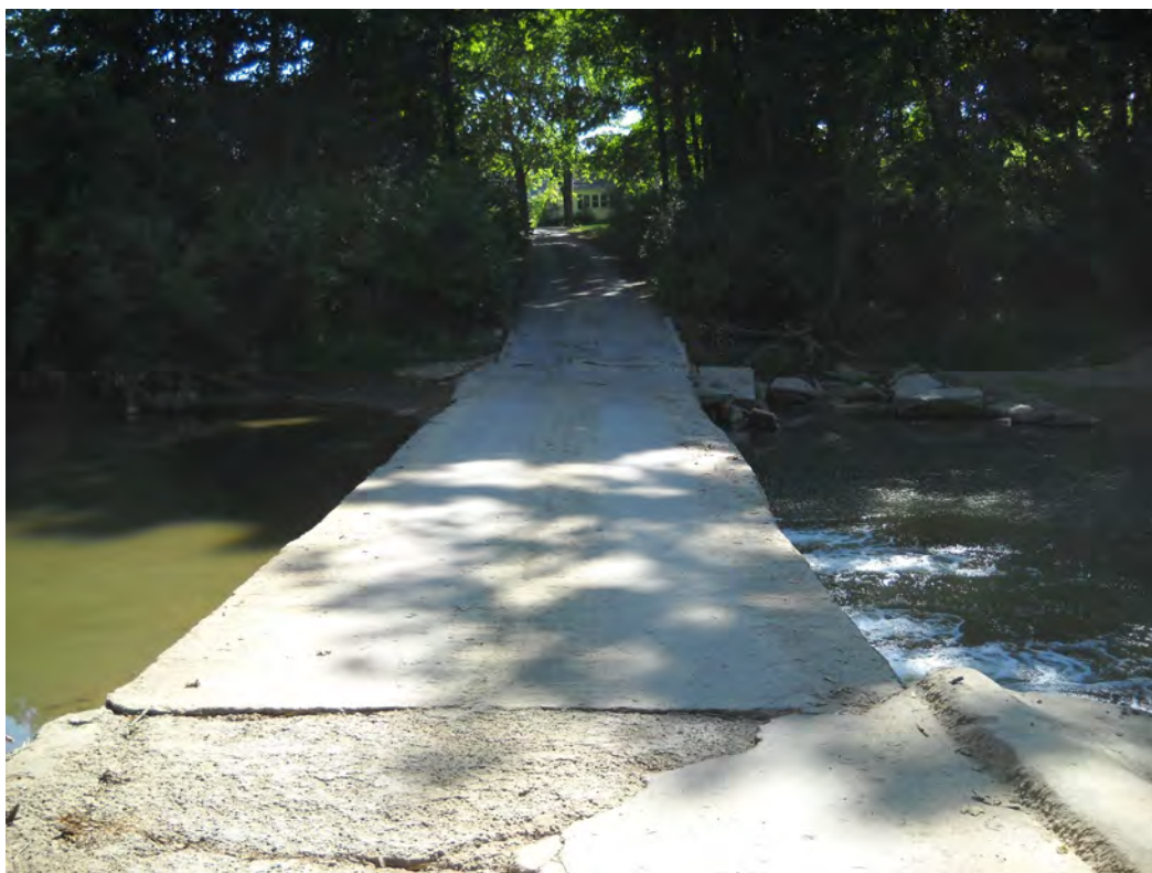
Looking east across low-water crossing
