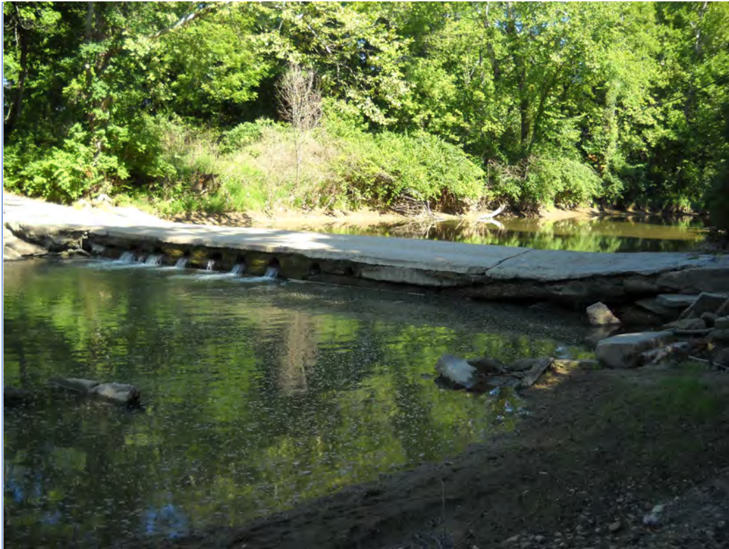
Sideview of downstream side of low-water crossing
