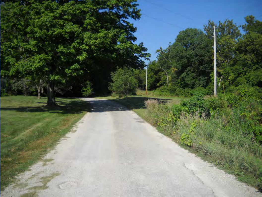
Near east end of project looking west along Staley Road
