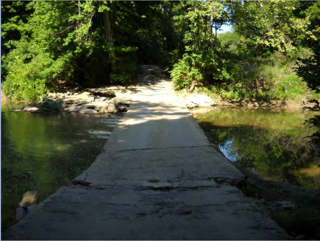
Looking west across low-water crossing
