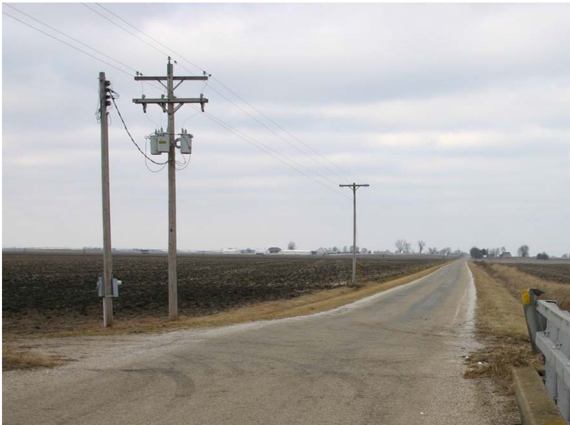
Photo 8 – TR 234 (3300E) - Looking North
