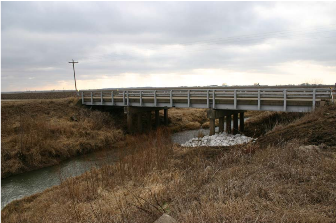
Photo 2 – Upstream (East Elevation of Existing Bridge) – Looking southwest
