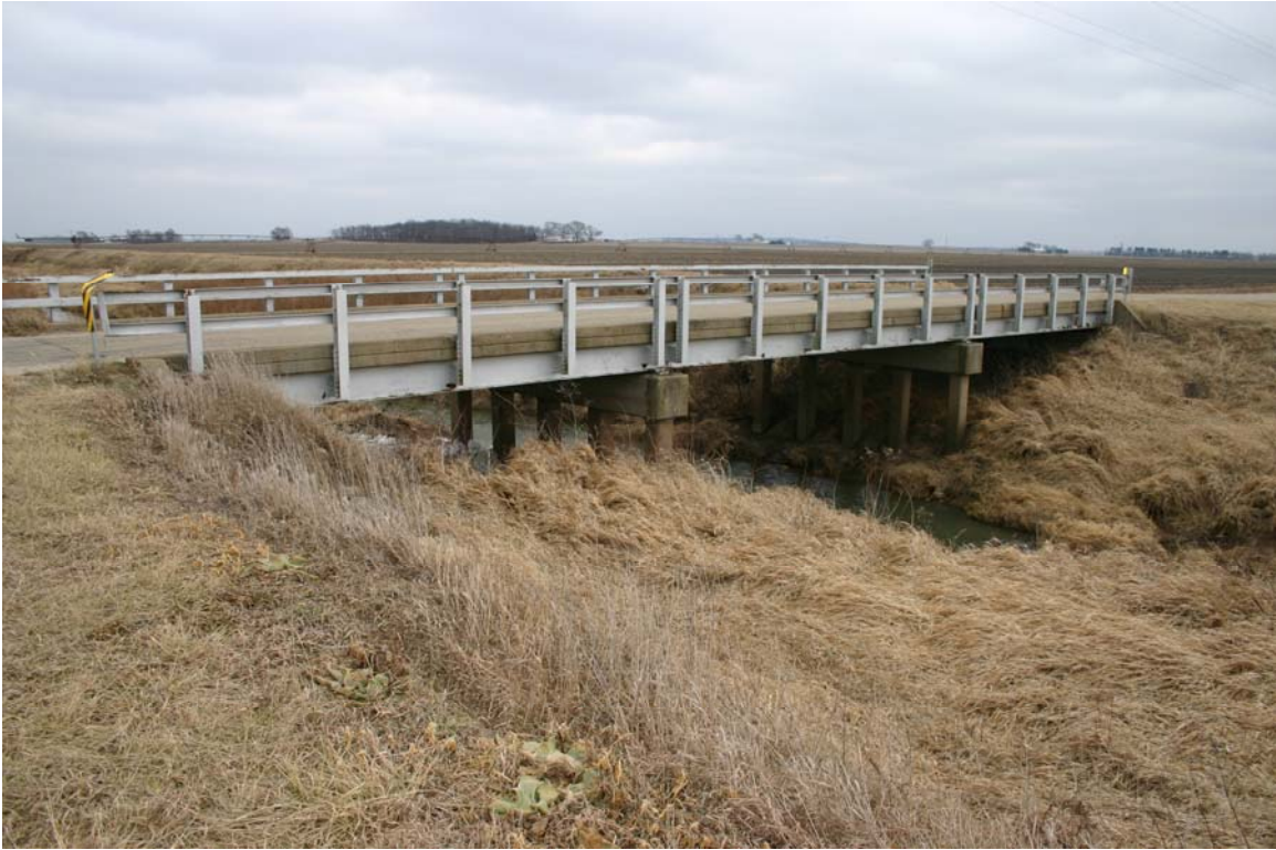
Photo 1 – Downstream (West Elevation of Existing Bridge) – Looking southeast
