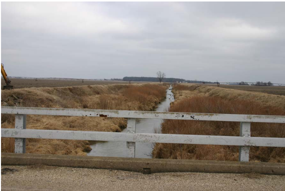
Photo 6 – Upstream channel - Looking east (upstream) from bridge
