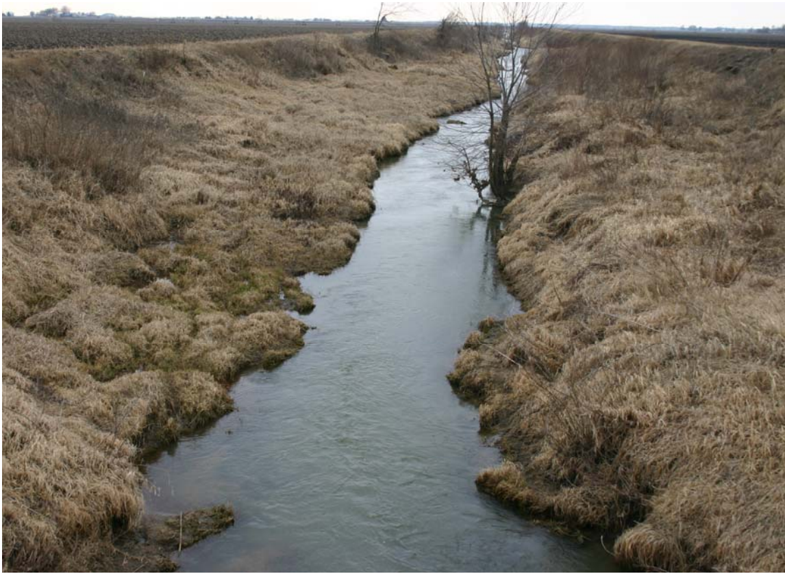
Photo 3 – Downstream channel - Looking West (DS)
