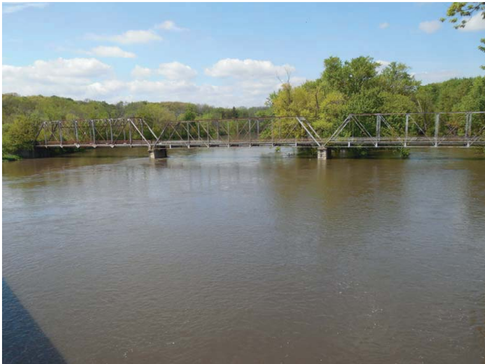
Photo 2 - Looking West across South Bridge Fascia
