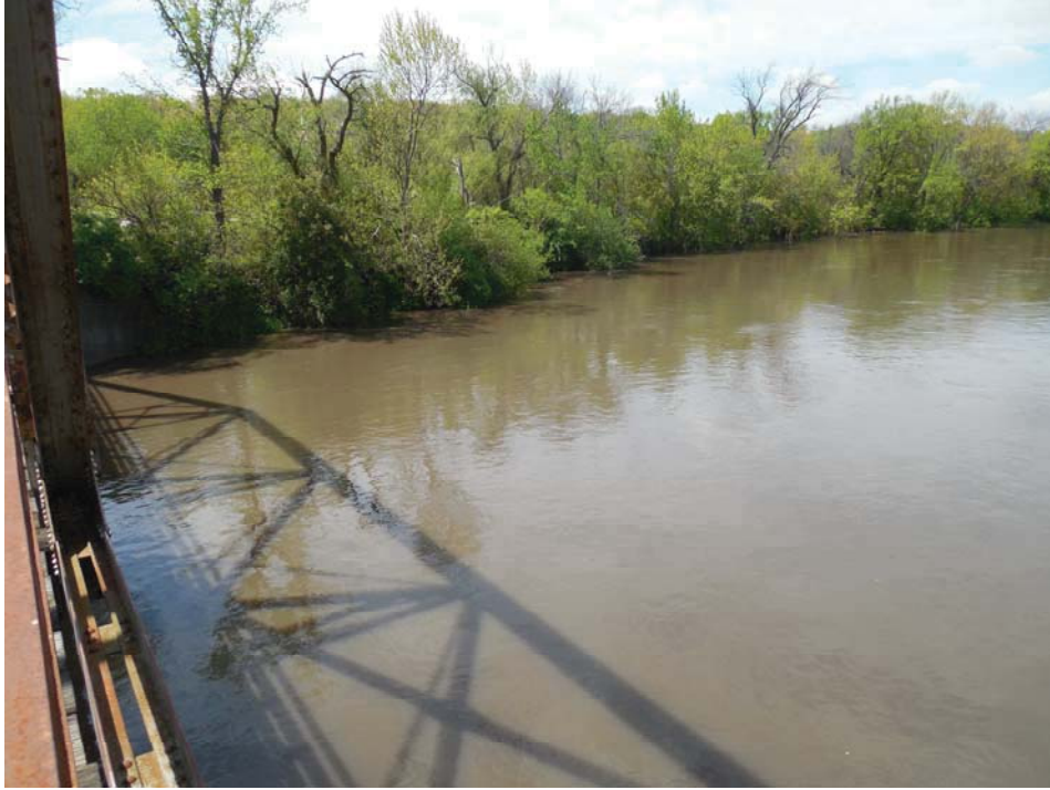
Photo 5 - Northwest from Center of Bridge
