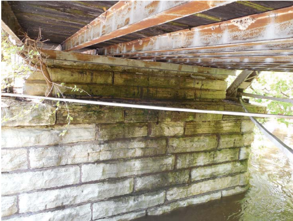
Photo 13 - East Side of East Pier
