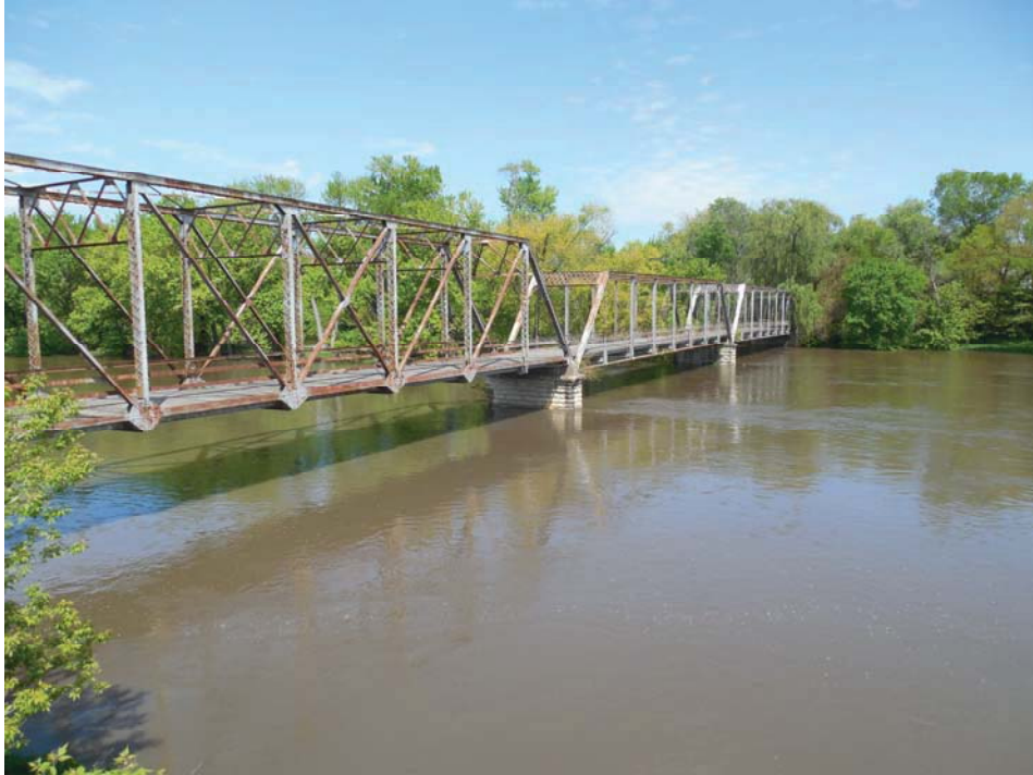
Photo 1 - Looking East across South Bridge Fascia
