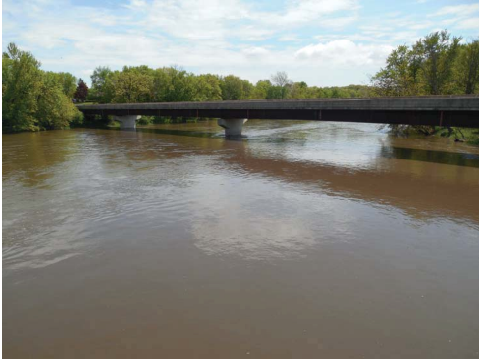
Photo 11 - South from Center of Bridge - Looking Downstream
