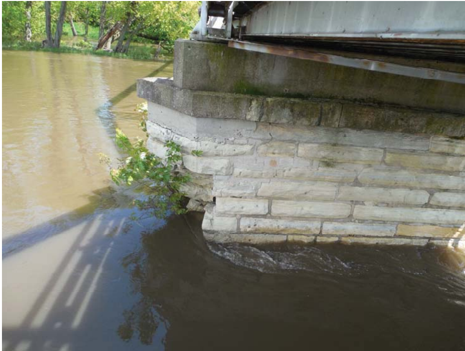
Photo 9 - Northwest Side of West Pier
