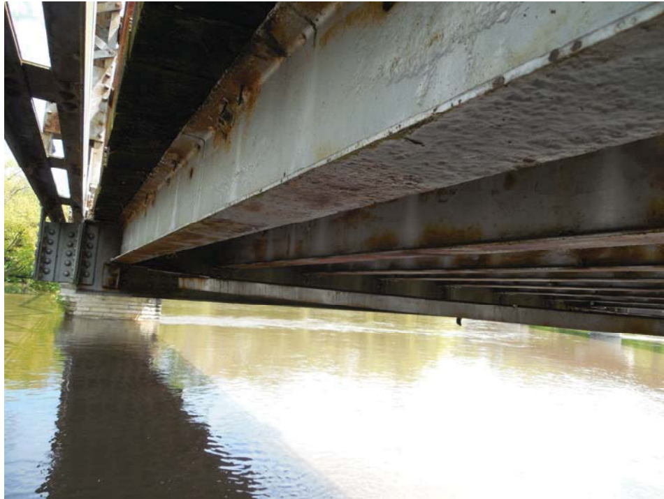
Photo 7 - Looking East at Beams under West Truss
