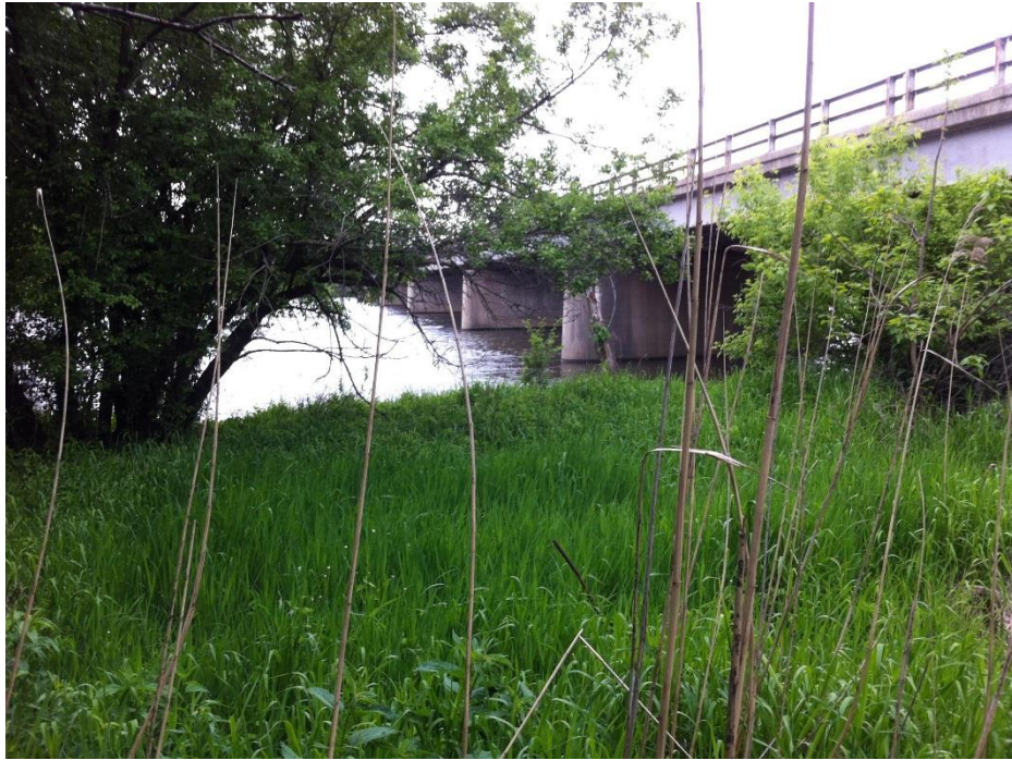
Northwest quadrant of the bridge, shoreline, and adjacent vegetation shown
