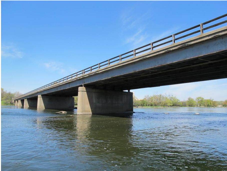
South side of bridge looking west across Des Plaines River
