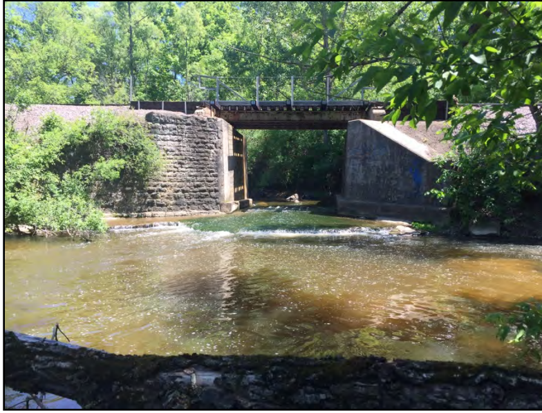
Image of site N002 looking upstream at the RR Trestle.
