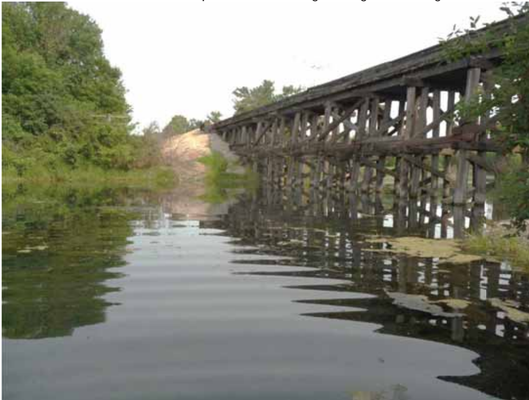
Plate 2. South side of the Freeport W 78.0 Bridge. Image is looking west.
