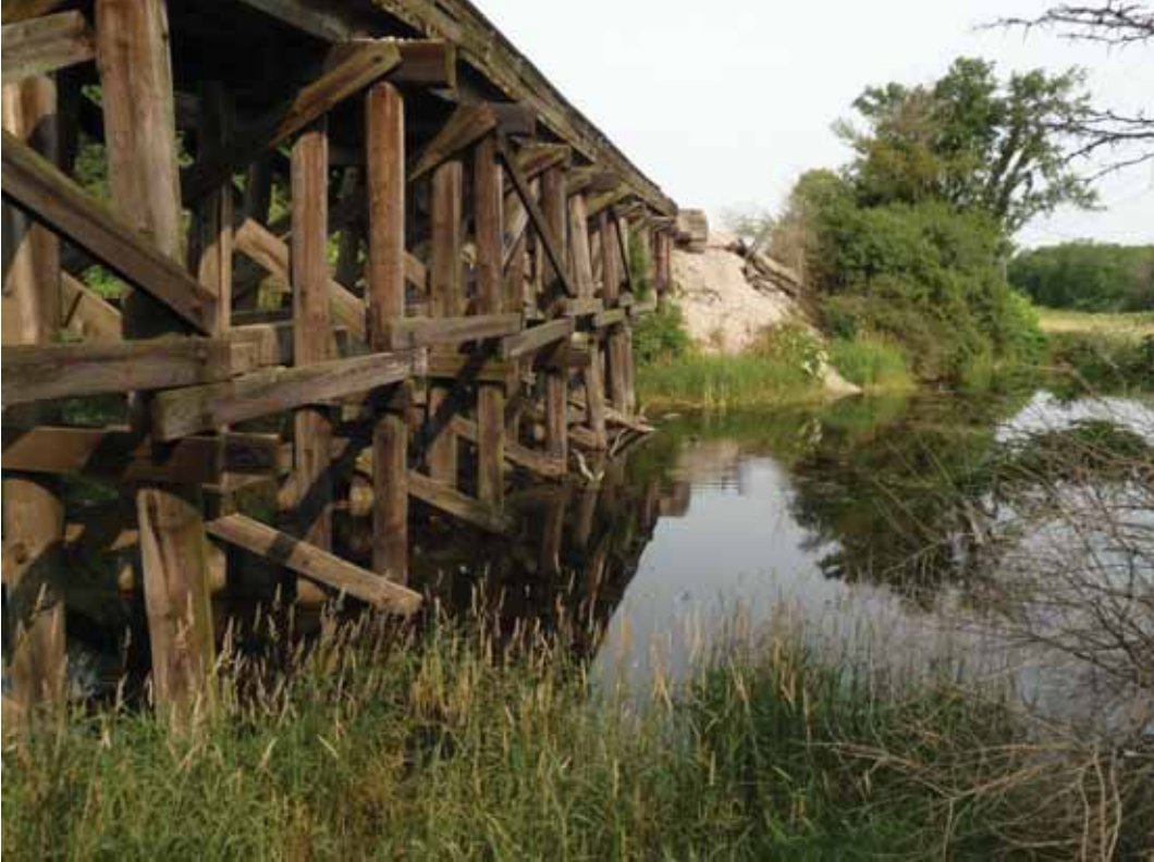
Plate 4. North side of the Freeport W 78.0 Bridge. Image is looking west.
