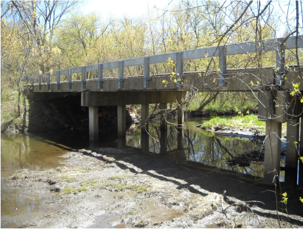
Subject bridge, facing southeast, spring 2015.
