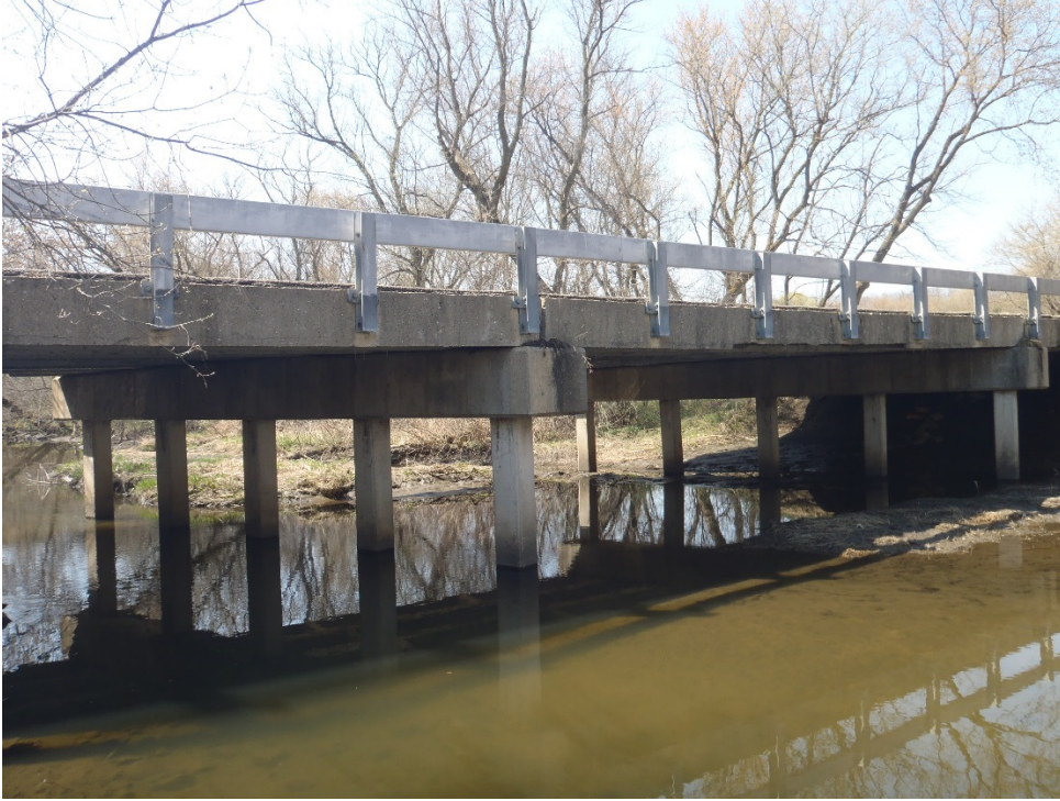
Subject bridge, facing southwest, spring 2015
