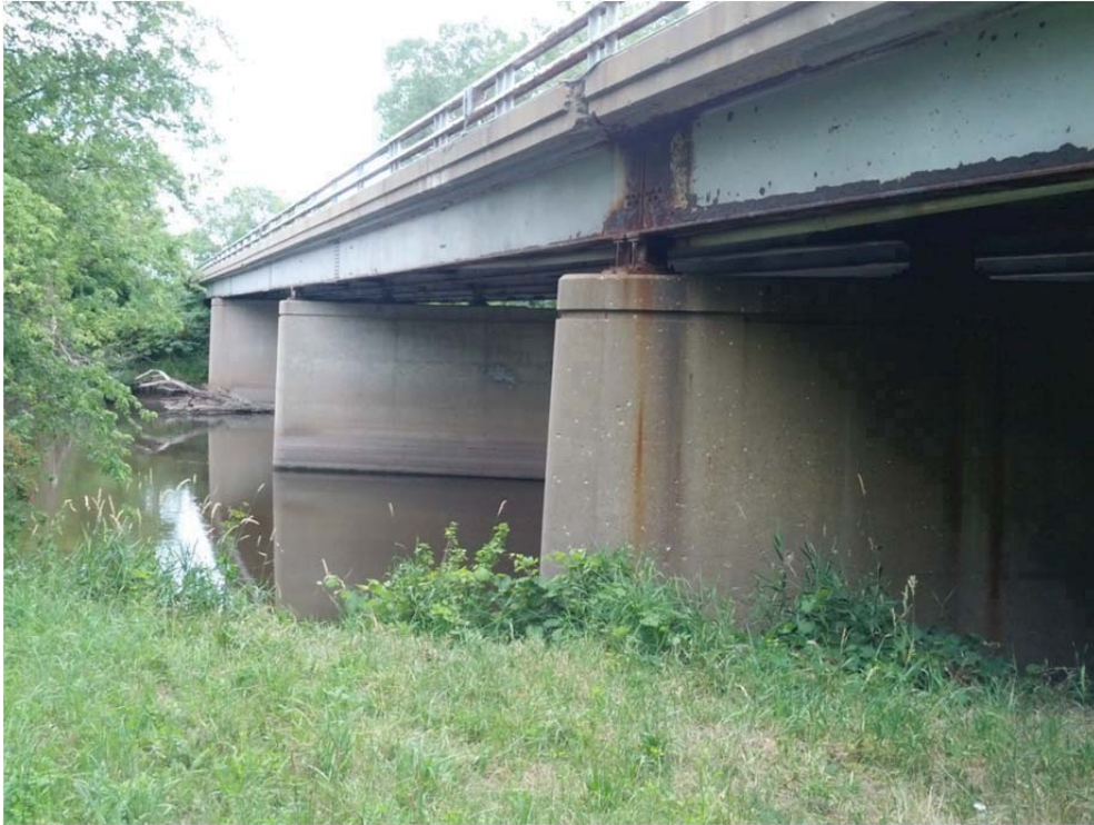
Pier 3 – South Elevation
