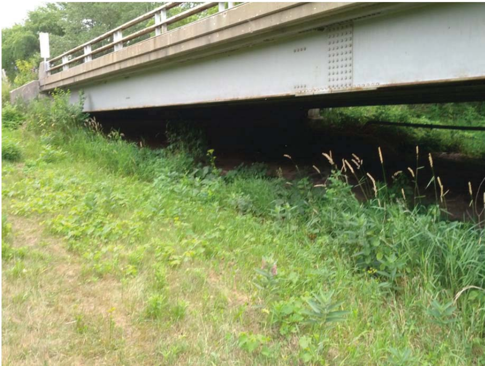
East Abutment Slope
