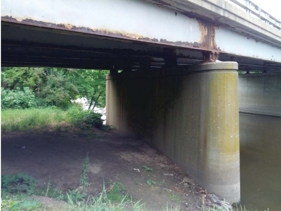
Pier 3 – North Elevation
