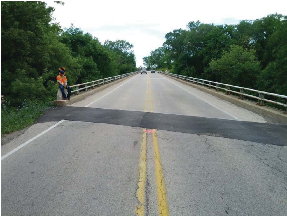
Looking West – East Abutment
