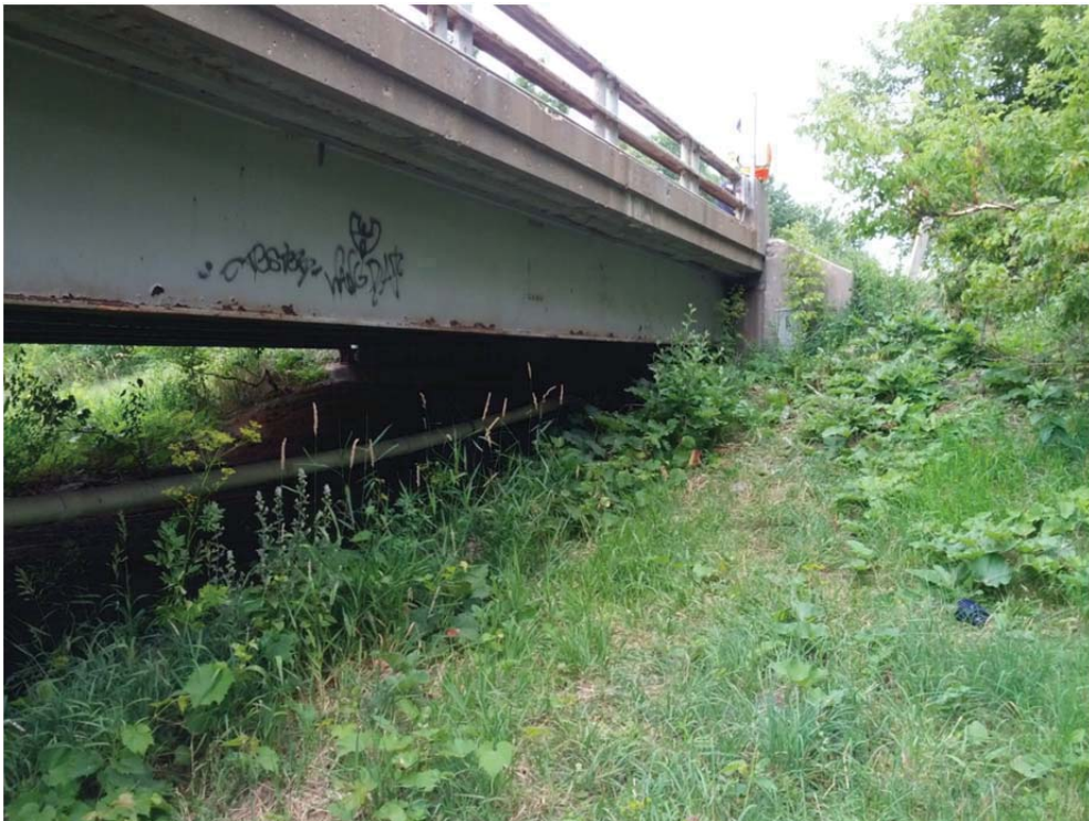
East Abutment Slope – South Elevation
