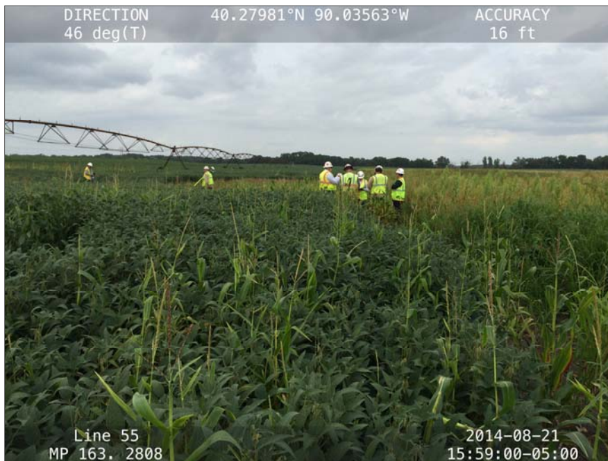
Facing northeast. Work area.
