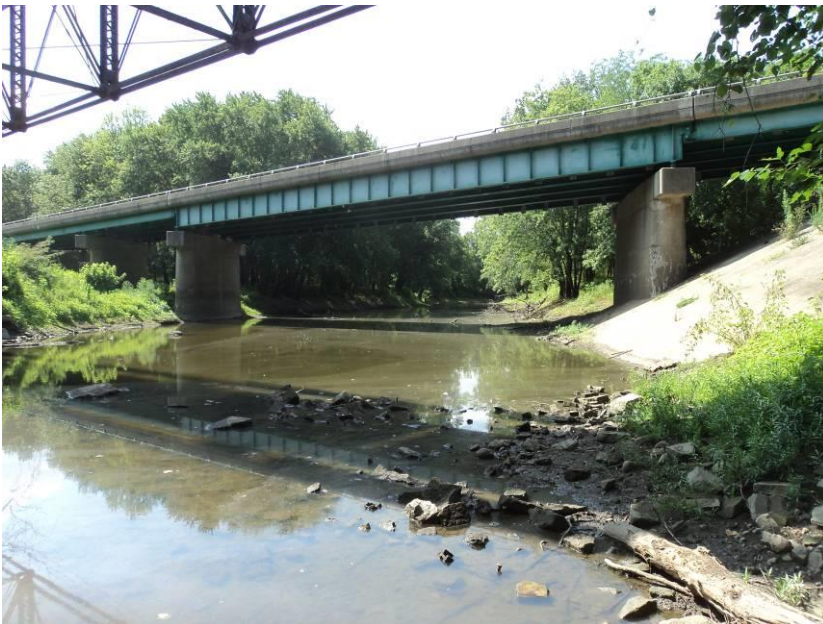
Looking south at IL 133 bridge from under abandoned railroad bridge. Photo taken July 16, 2012.
